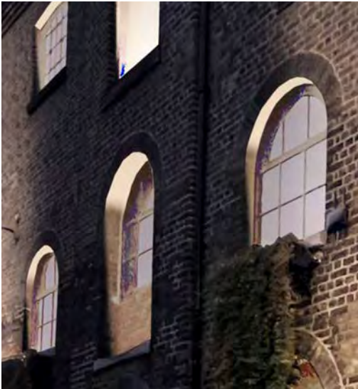
Proposed lighting effect using diffused linear LED profile to typical external windows.
