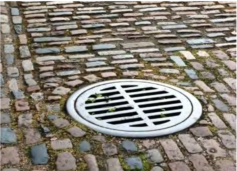
Covering for skylight that provides ventilation and natural light for the underground tunnels that can be found scattered across Camden Market grounds.
