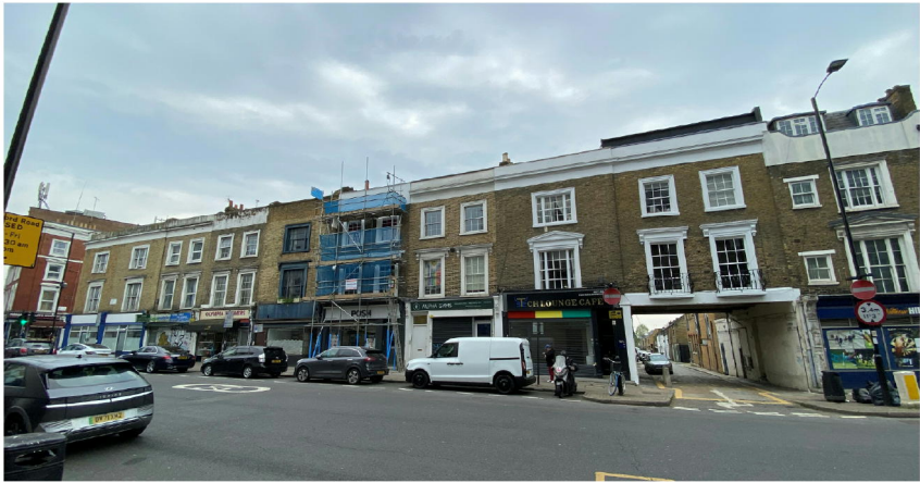
View of current terrace streetscape.
