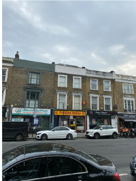
View of roof extension to no. 177.
