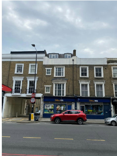
View of roof extension to no. 169.
