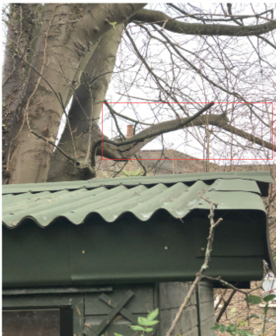
Hazard Beam split limb on the north side of T2 at approx. 4m.
