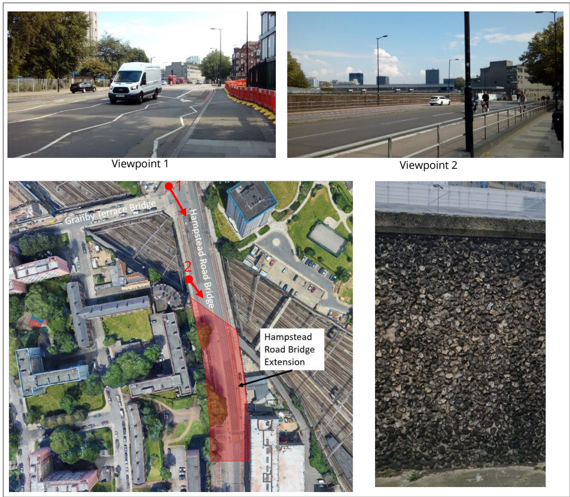
Figure 2 Street level and aerial views of the existing Hampstead Road Bridge. Bottom right: Existing 1.65 metre parapet located along the outer extents of the existing Hampstead Road Bridge (Source: Google Earth). Red area illustrates location of the Hampstead Road Bridge Extension (indicative only).
