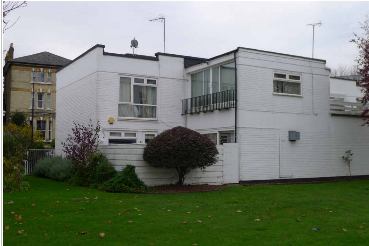
REAR ELEVATION FACING NORTH
