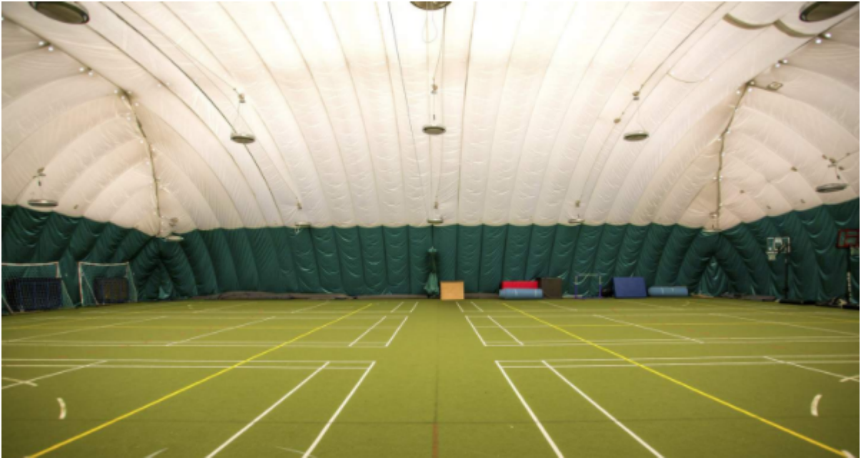
4. Inside of the dome
