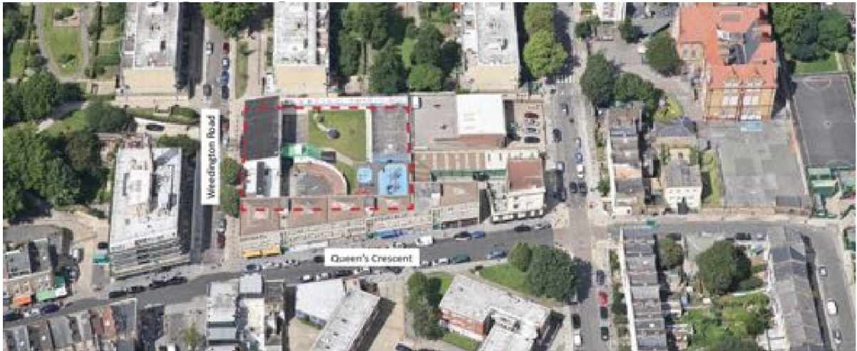
1. Site prior to installation of dome ref. 2013/5667/P
