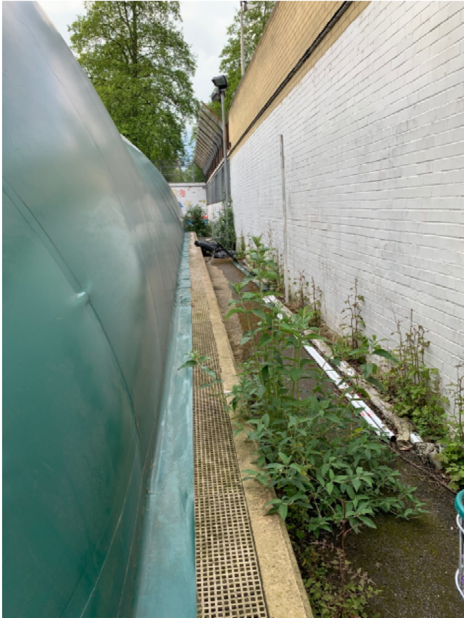
3. Drainage canal as existing
