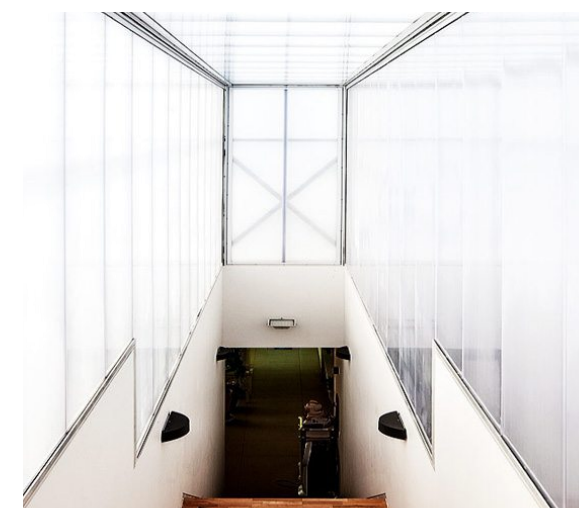
03. Example of feature polycarbonate wall panel on SFS with concealed back lighting.
