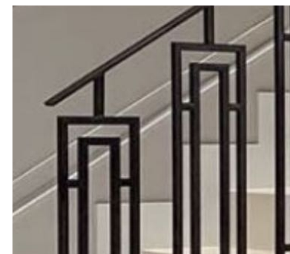
05. Art Deco inspired handrails for stair central handrail. Bolt fixed at floor level.
