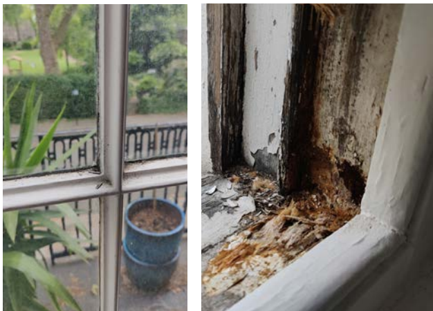
Existing window bars and visible frame deterioration
