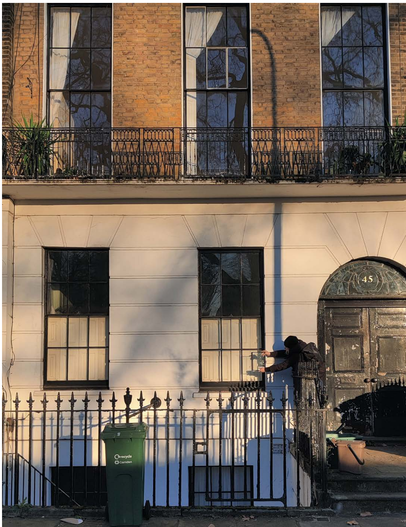
House 45 - comparison of model of proposed window bar held against existing
