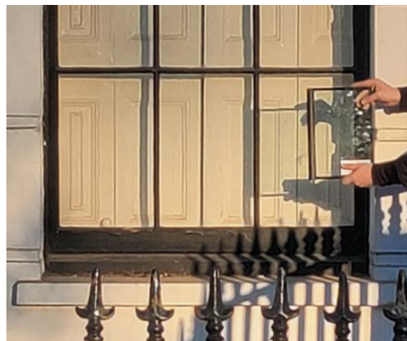
House 45 - model of proposed window bar against existing
