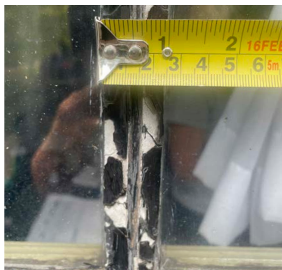
Existing example showing external width of 24mm - varies
