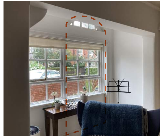
Fig. 11. Openings don't reflect original spaces, e.g. historic stable door
