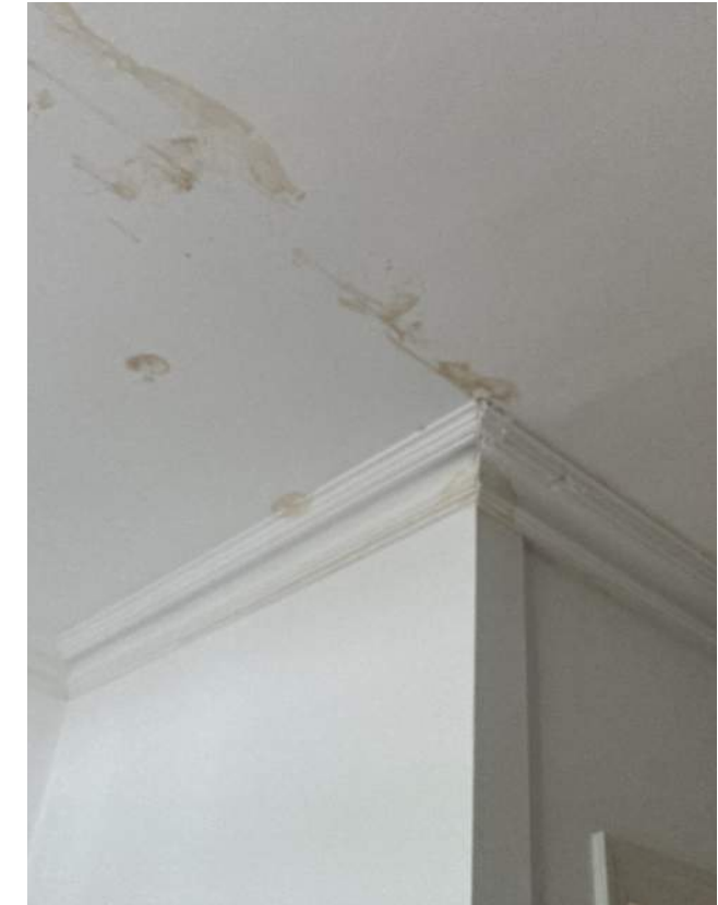
Fig. 20. Water damage
