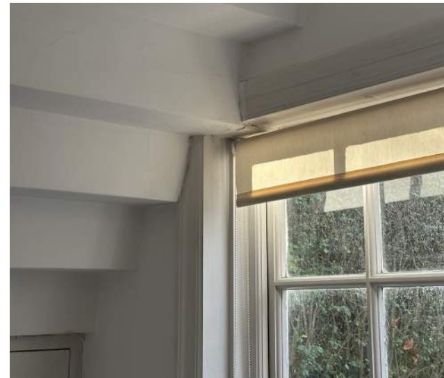
Fig. 10. Messy connections to widened window opening
