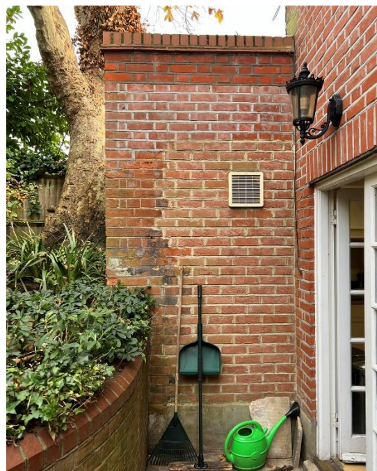
Photograph 4 – Side elevation of rear part of building
