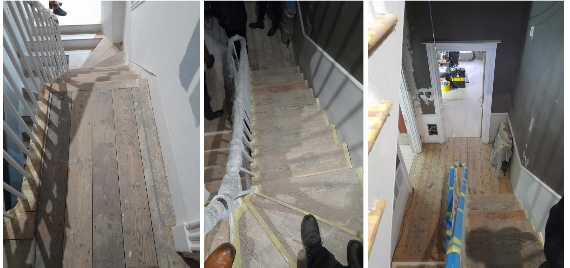
Timber stairs and floorboards at landing levels in the process of being cleaned and repaired.
