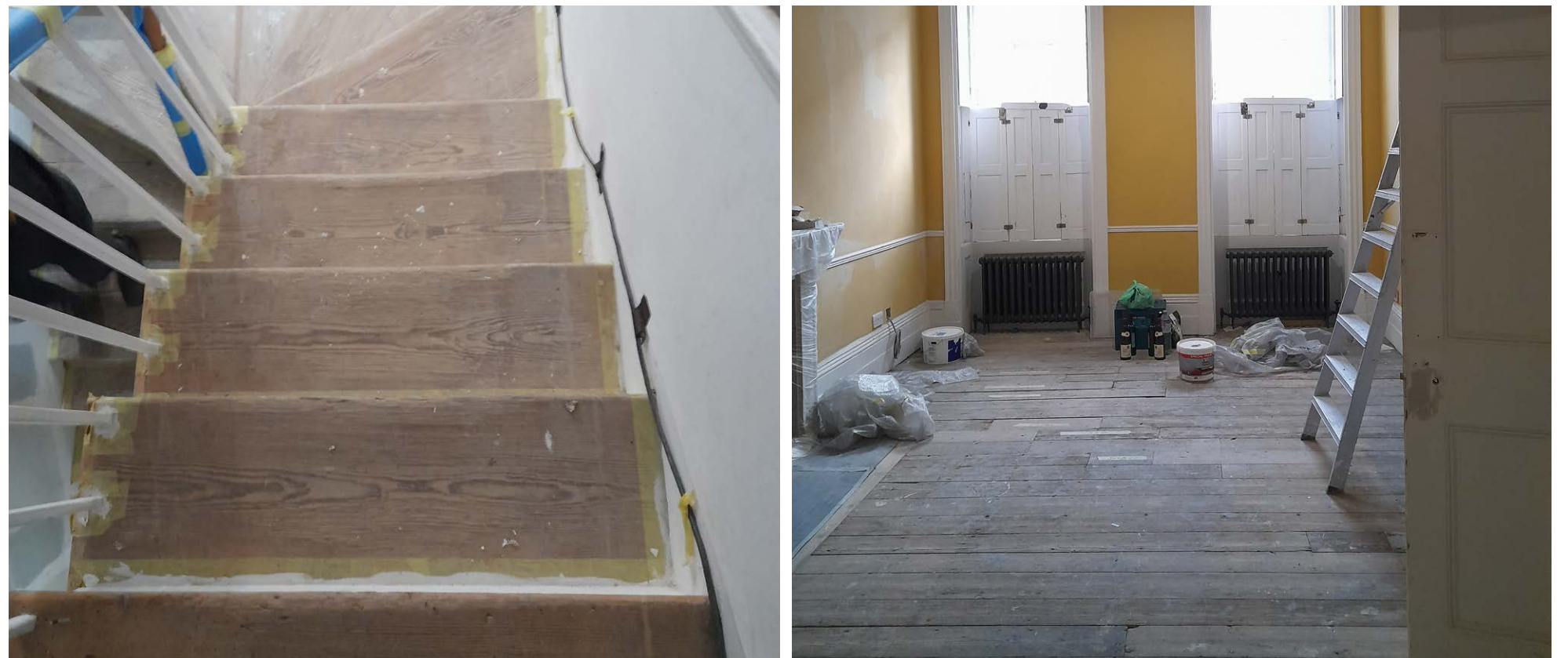
Timber stairs and floorboards in ground floor front room in the process of being cleaned and repaired.
