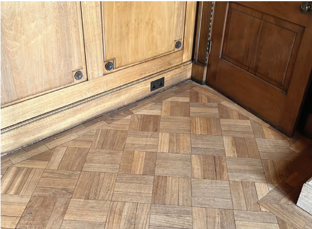
Heritage Rooms - Typical skirting power socket (Photo C)
