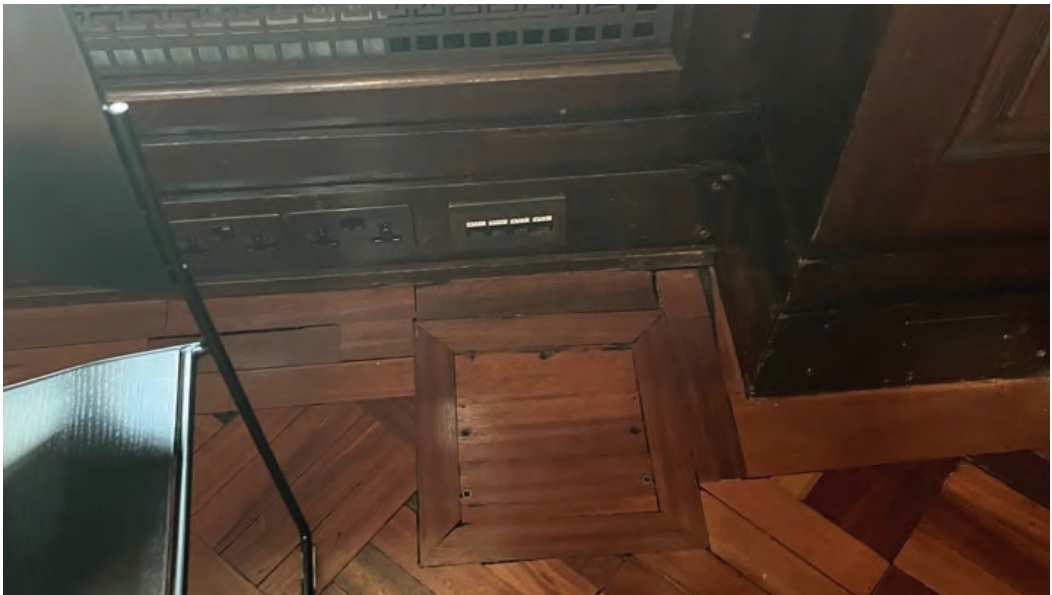
Heritage Rooms - Original floor box & skirting power and data (Photo B)
