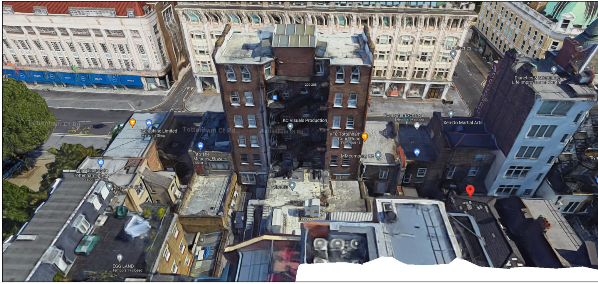
PHOTO IMAGE INDICATES EXISTING REAR ELEVATION
