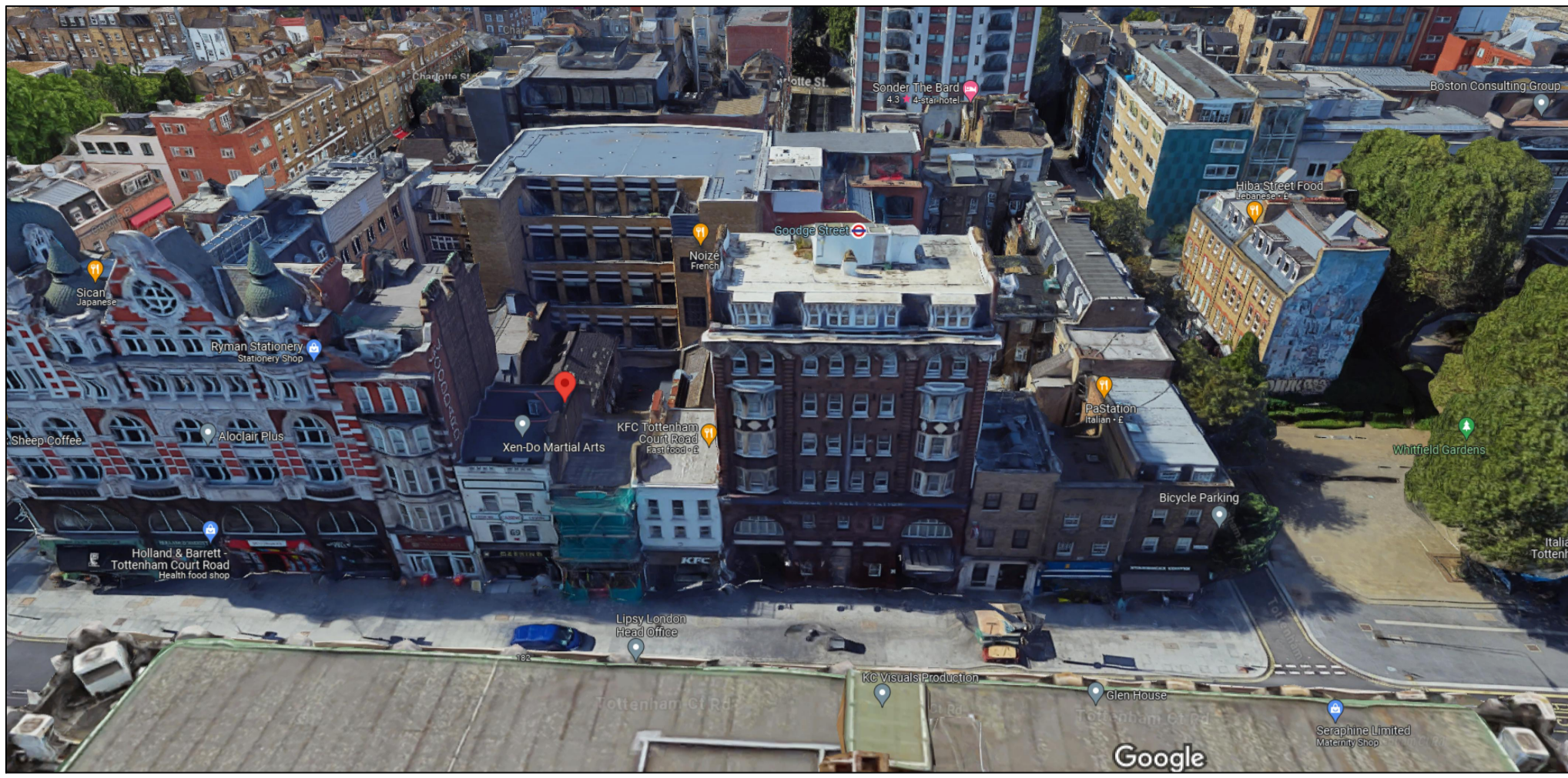
PHOTO IMAGE INDICATES EXISTING FRONT ELEVATION FACING TOTTENHAM COURT ROAD
