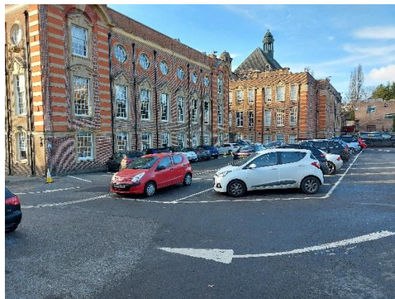
Plate 3: Main School Building
