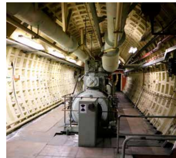
Pre-cast concrete lining
