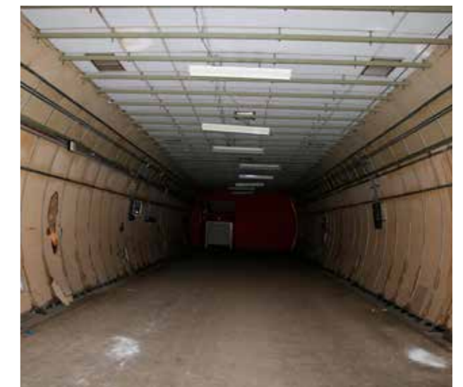
Laminate lining ( inside pre-cast concrete )
