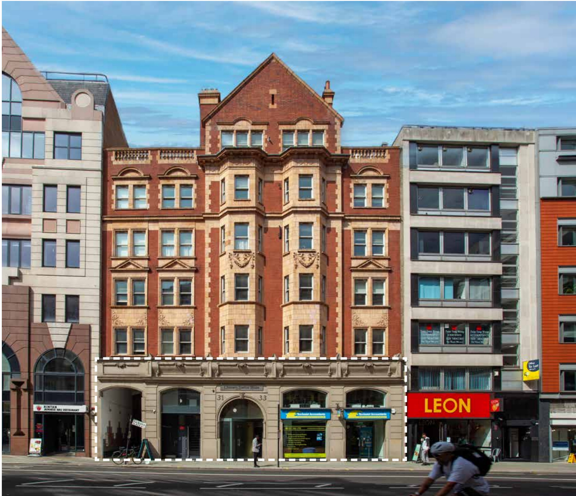
Figure 124. Current High Holborn elevation (30-31 High Holborn) Dotted white line indicates scope of facade included in the Proposed Scheme
