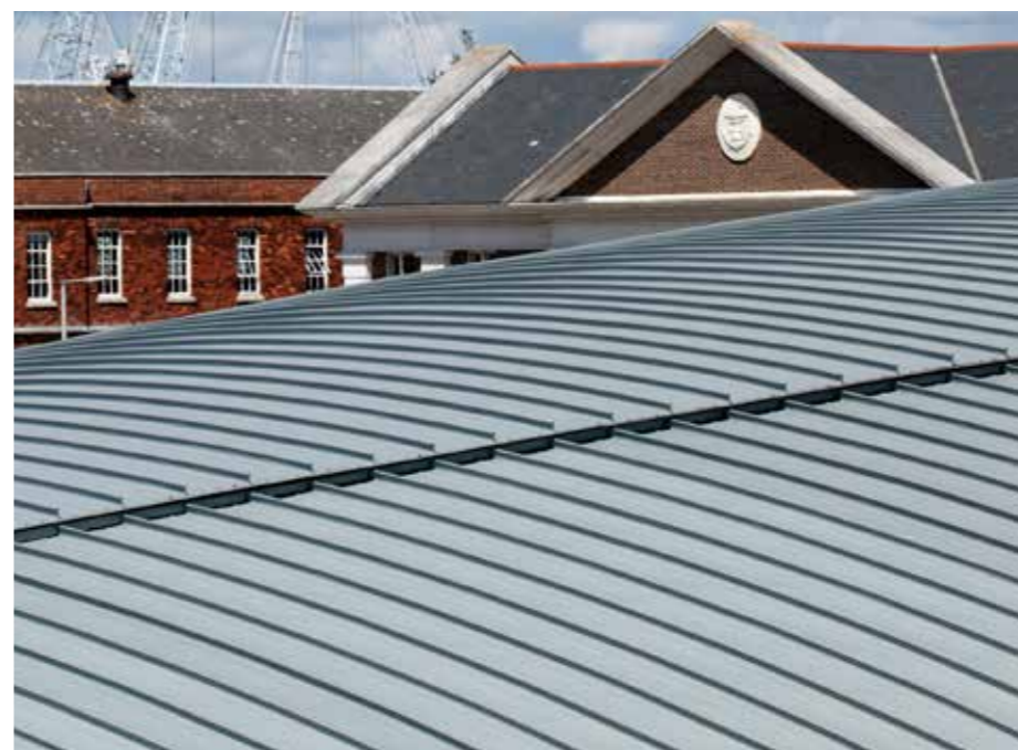
Zinc Standing Seam Roof / Cladding
