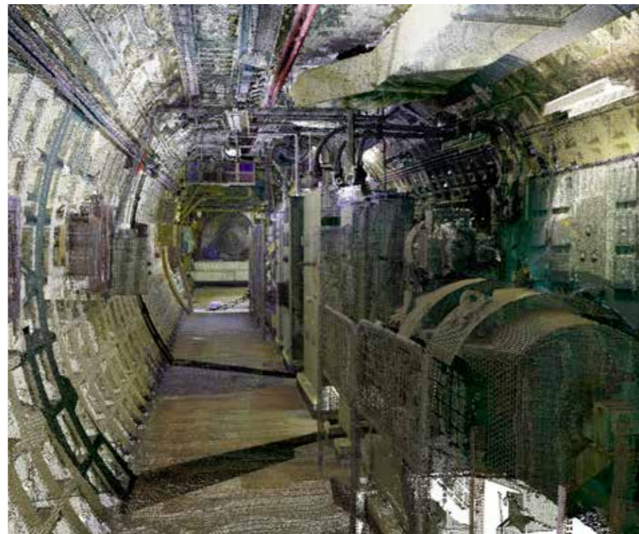
Point cloud extract - North Street East
