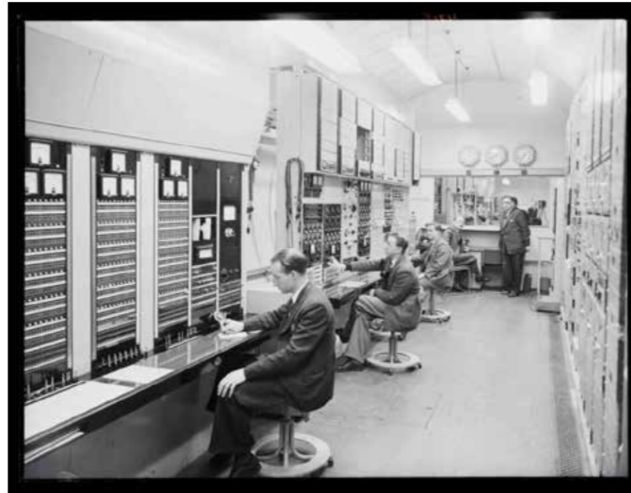
Figure 16. One of the telephone exchange rooms in the Kingsway Tunnels
