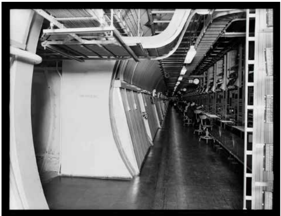
Figure 20. British Telecom archive images showing the interior of Kingsway Tunnels
