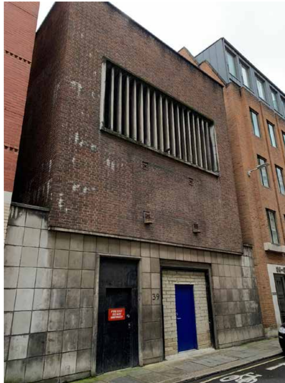
Figure 4.3 Photo of No. 39 Furnival Street
