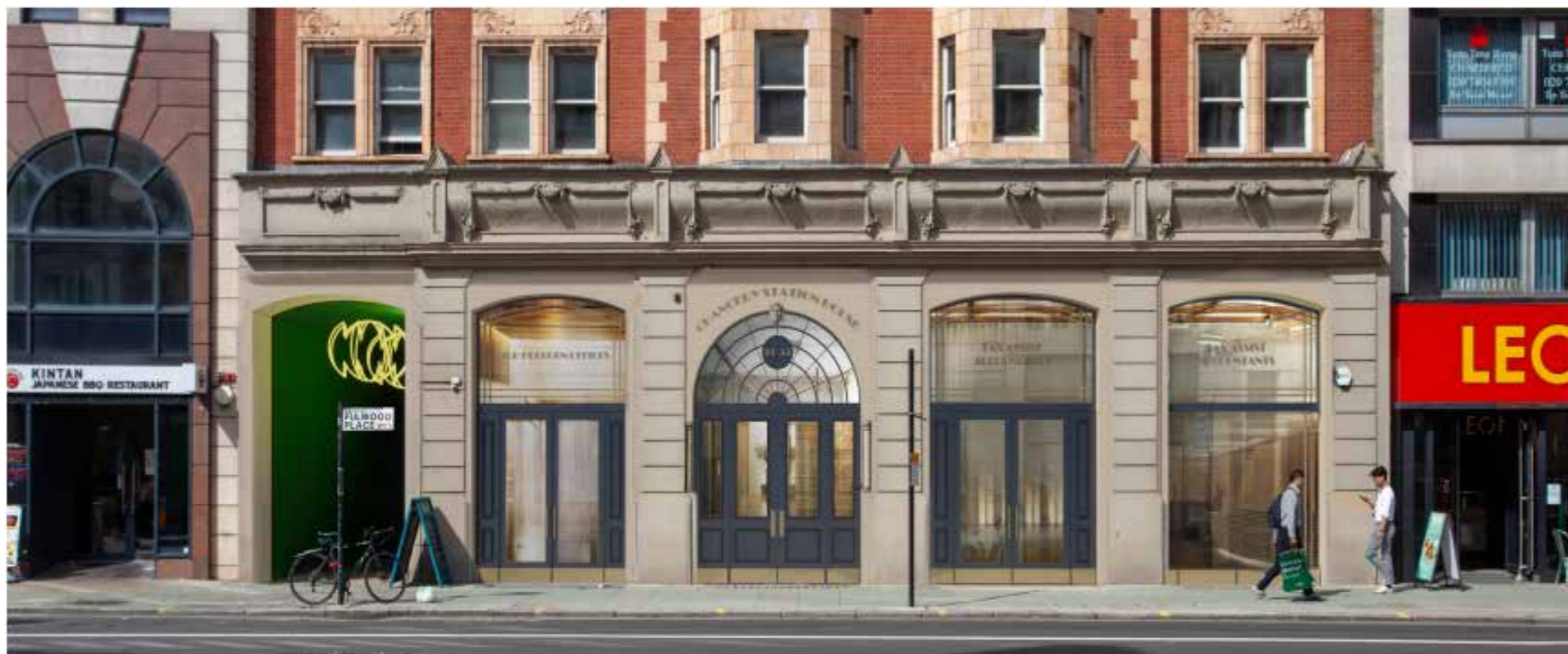
Figure 6.4 Improvements to ground floor frontage of 31–33 High Holborn (Source: Wilkinson Eyre Architects).
