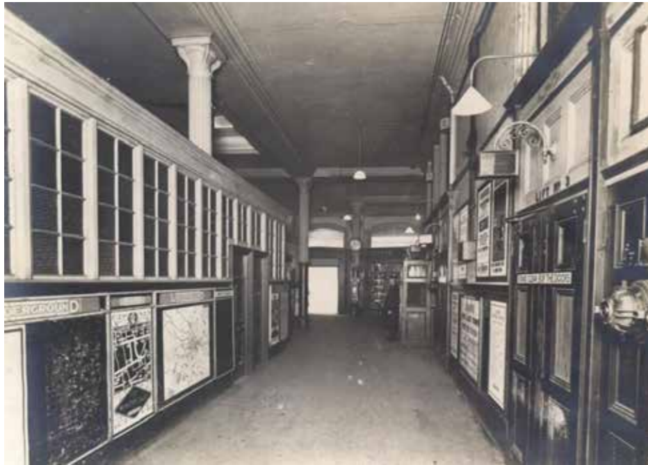
Figure 4.8 Interior of Chancery Lane ticket hall at No. 31-33 High Holborn, 1928 (source: London Transport Museum)
