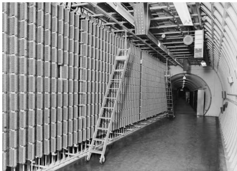
Figure 3.8 Main Distribution Frame, 1957 (source: BT Archive)
