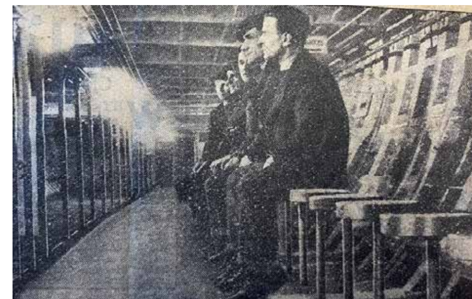
Figure 3.5 Interior of the Chancery Lane deep level shelter, 1946.
