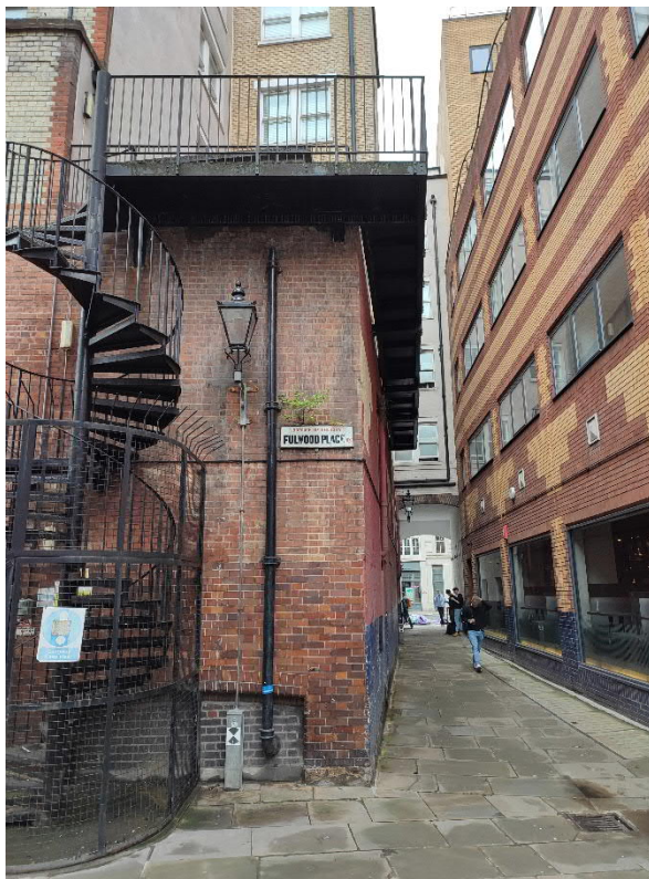
Photo 2: View from Fulwood Place down to High Holborn down the site of the Fulwood Place Site building.
