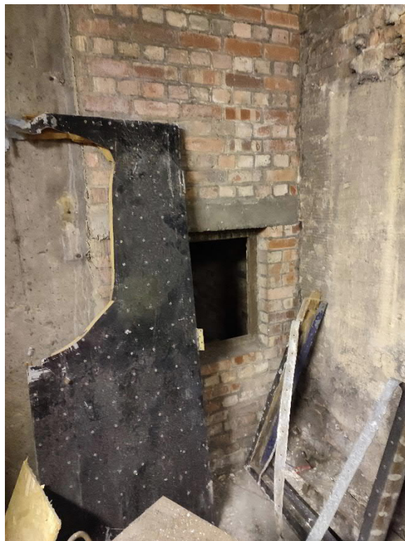
Photo 10: Photo of the south interior wall of the shaft ventilation room.
