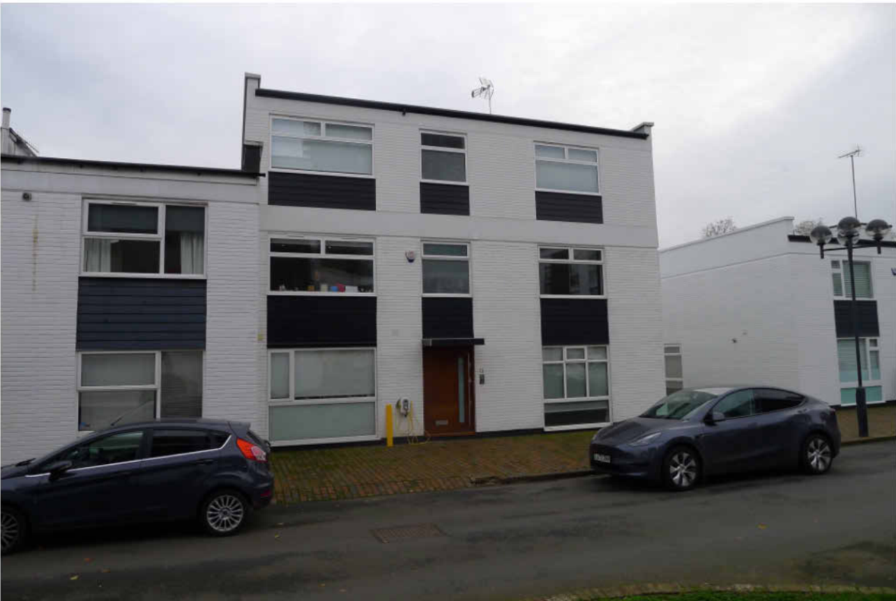
Number 13 Hawtrey Road, Alternative front door design, two opening top vents to most windows, glazing floor to ceiling ground floor.
