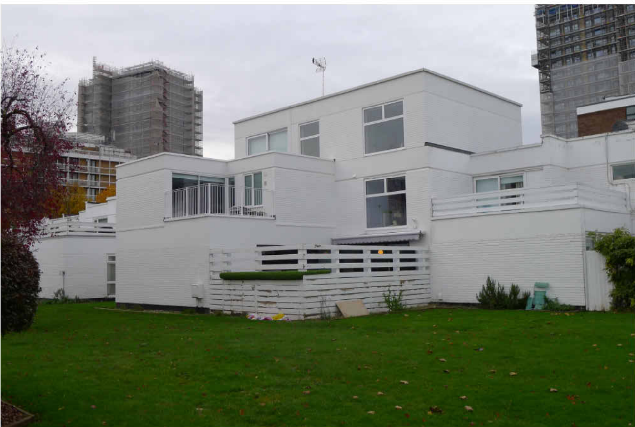
Number 13 Hawtrey Road, Rear elevation. Windows with two opening top vents, floor to ceiling windows to 1st and 2nd floors.
