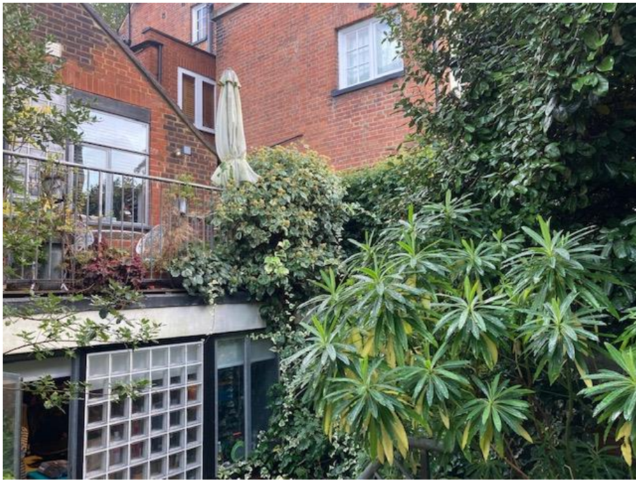
3. Existing rear elevation (basement room and ground floor level) and shared boundary with No 8. Hollycroft Avenue
