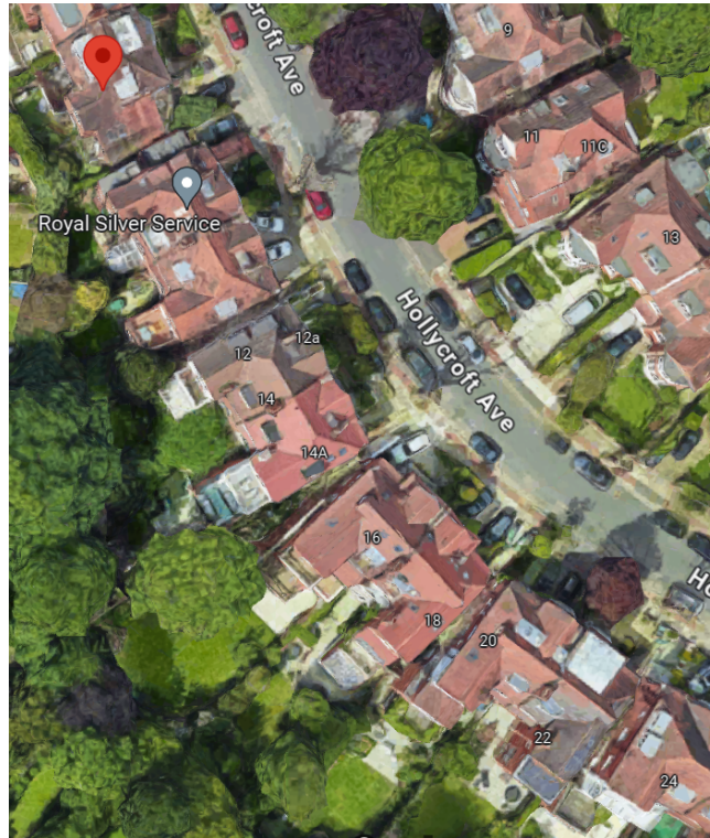
Fig 1. Ariel view of similar rear extensions at multiple neighbouring properties on Hollycroft Avenue
