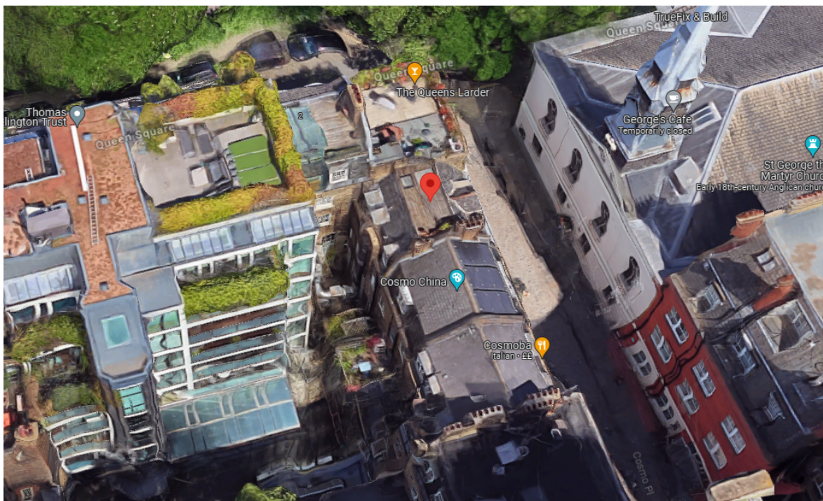
Photo 2 (above): Aerial perspective view (source: Google 3D)
