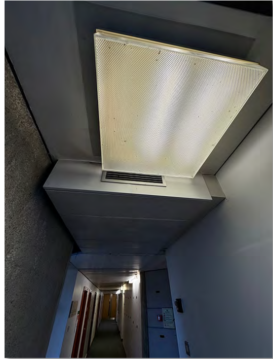
IMG_0755 Bulkhead within corridor dead end zone
