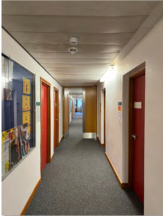
IMG_0749 Mid corridor 1½ leaf fire door
