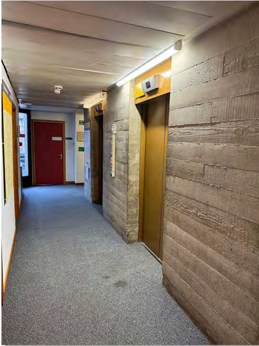
IMG_0724 Area outside lift doors
