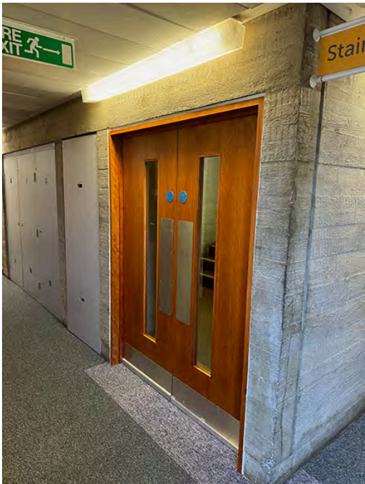
IMG_0744 Doors to Stair 4
