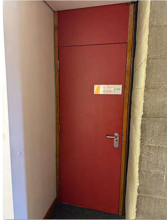
IMG_0734 Later addition plastic laminate faced door and over panel to Room P503
