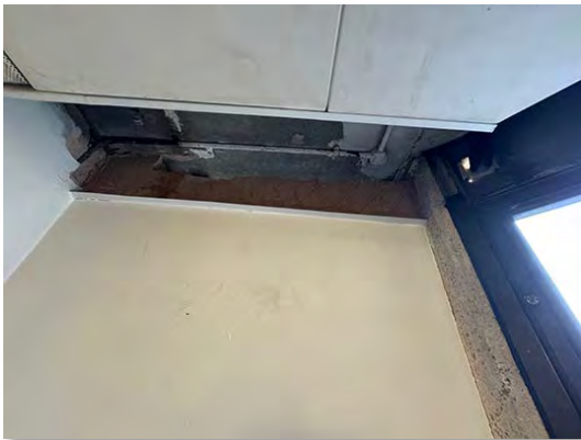
IMG_0727 Area of ceiling slab above suspended ceiling
