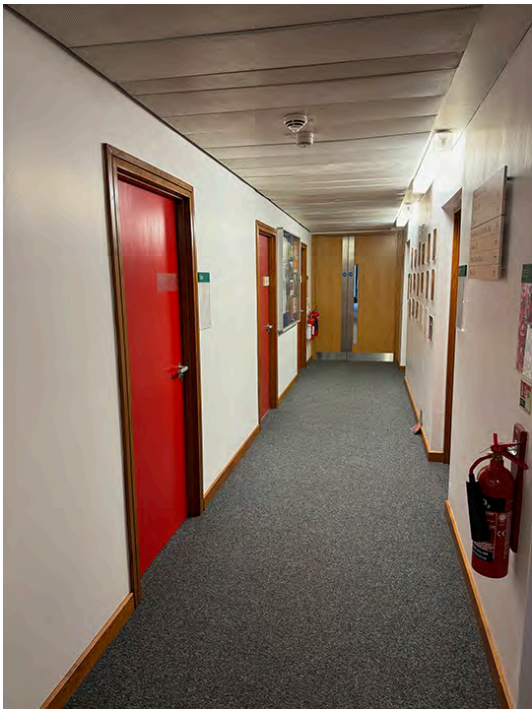
IMG_0735 Mid corridor 1½ leaf fire door
