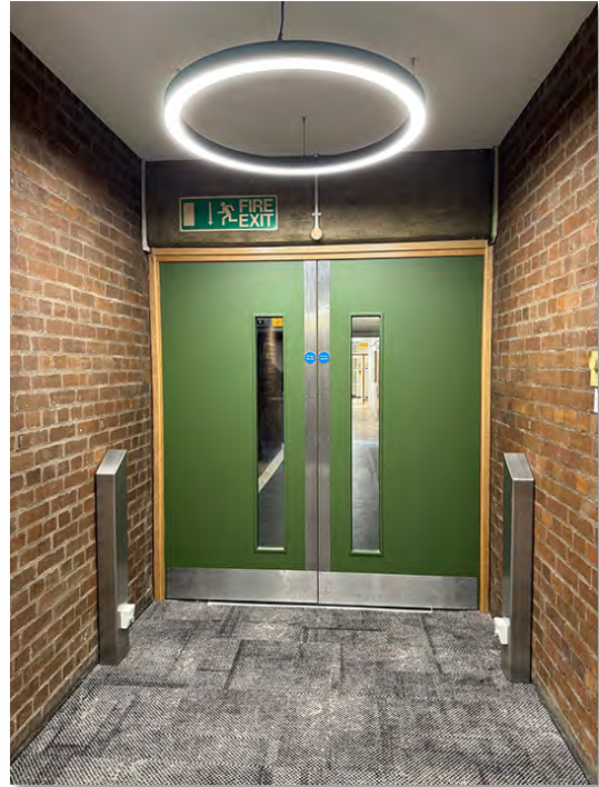
IMG_1061 Vinyl wrapped fire doors at head of Link Bridge
