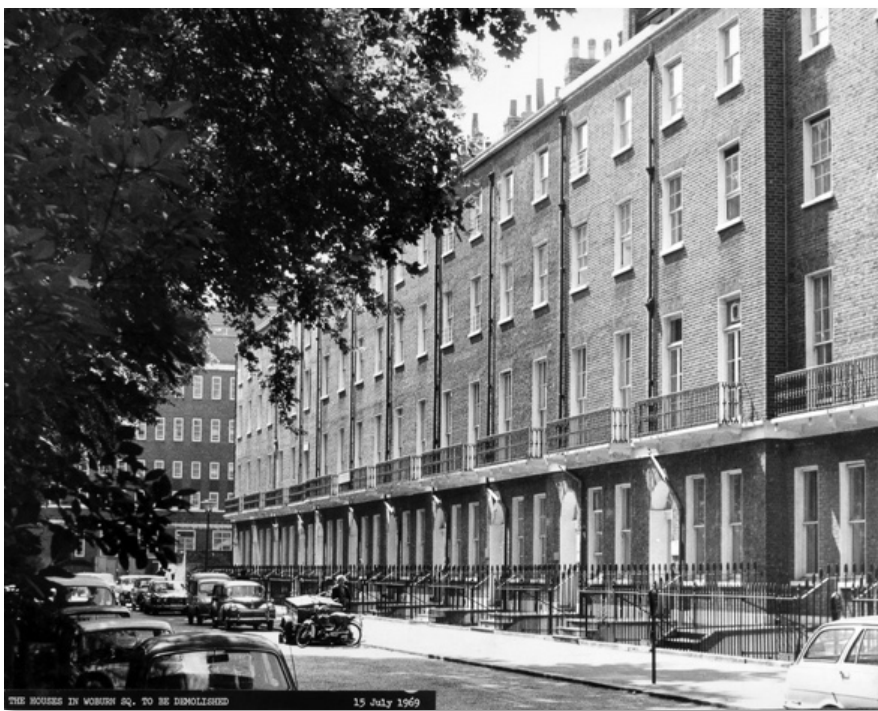
Woburn Square pre demolition 1969
