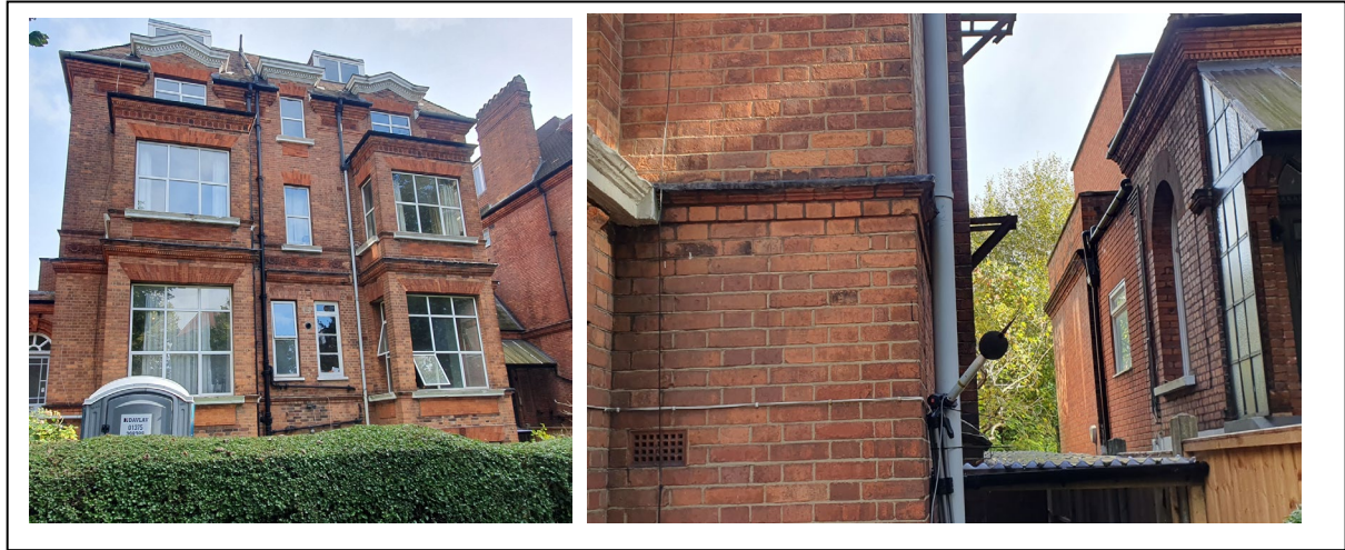
Figure 3: Site Location Measurement Pictures
