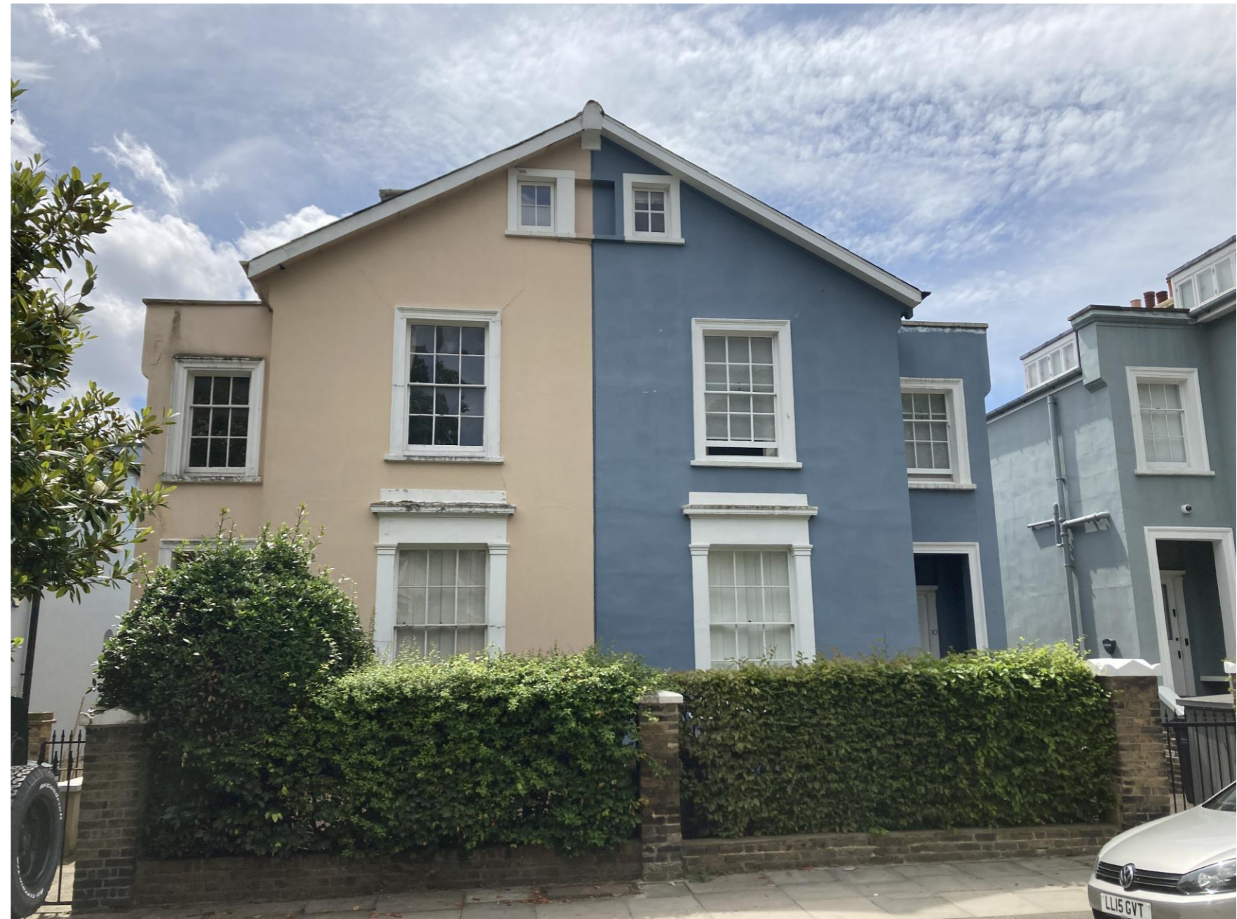
Figure 1: Front Elevation of Property
