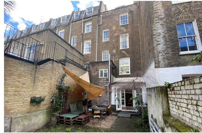
fig 3.1 Photograph - Existing Rear Elevation
