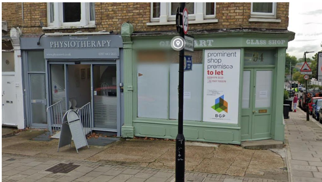
Lightwells, ramped access and railings at no. 96 Mill Lane
