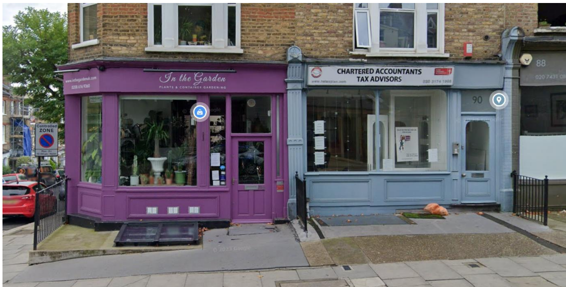
Lightwells and railings at nos. 92 and 90 Mill Lane
