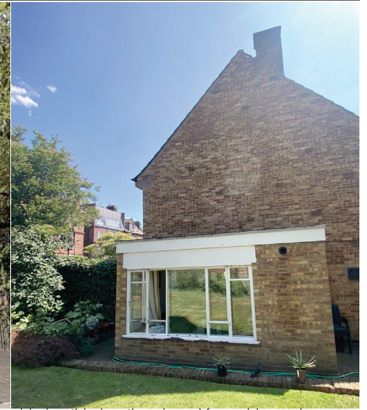
side (north) elevation viewed from side garden
