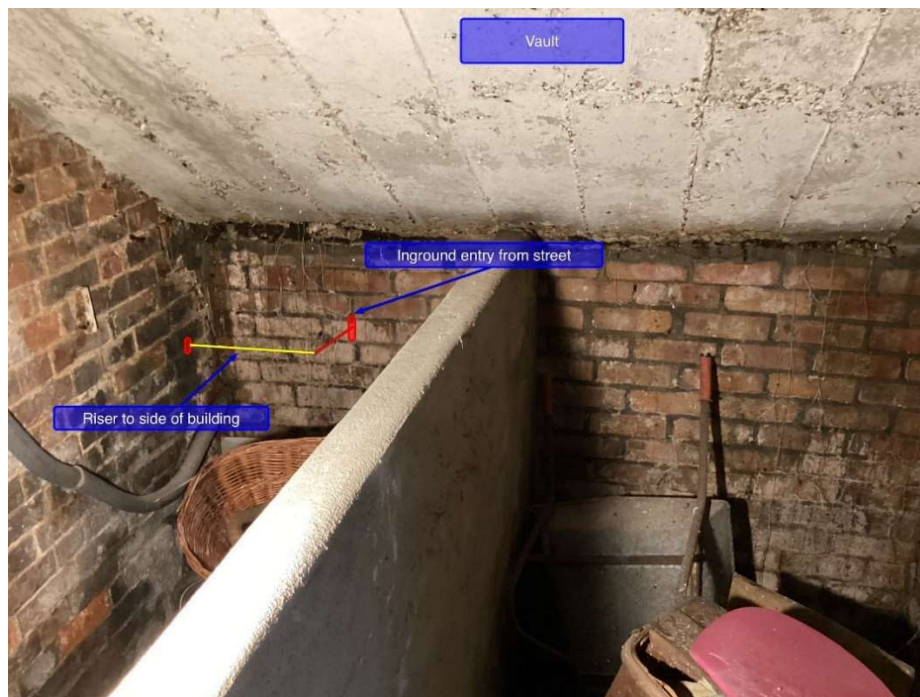
Figure 1 Proposed pipework to basement vault areas.
