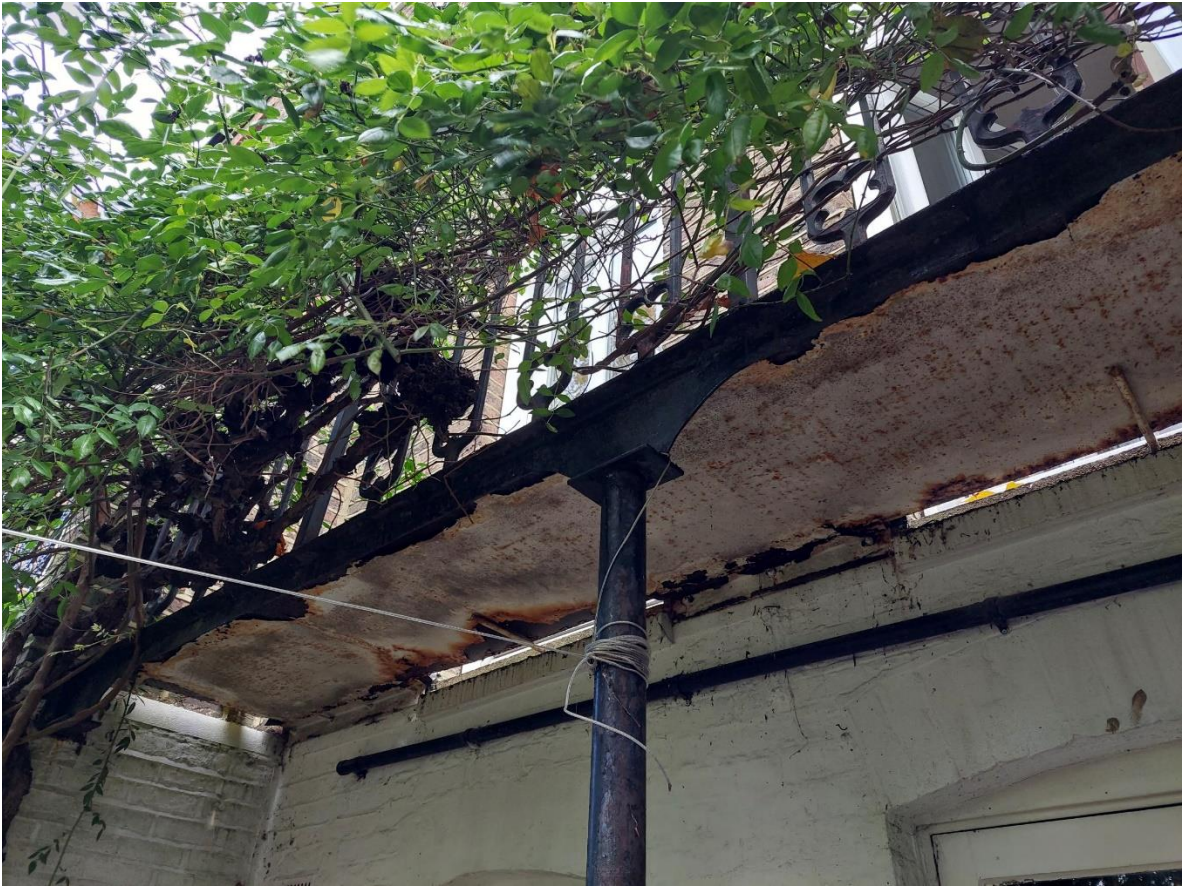
Figure 3: Existing Condition of Balcony.
