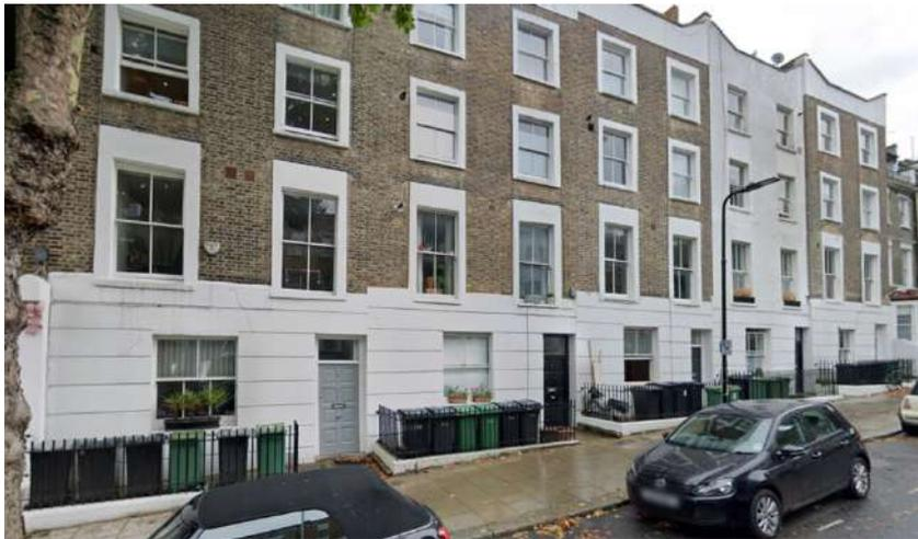
Figure 2 [above]: View of no.3 to no.7 Ainger Road showing the infilled front lightwells
