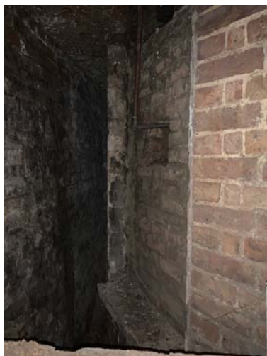
Figure 11: Existing Rear Well with blocked window openings and concrete slab above.
