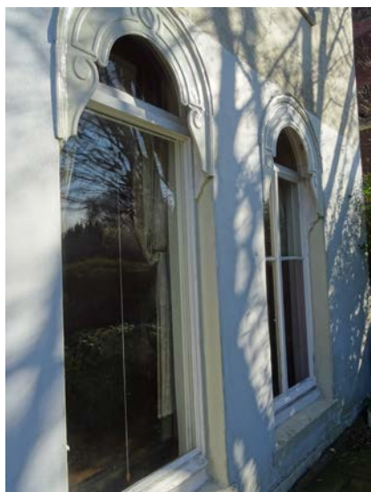
Figure 17: Fixed window to patio and bonnet blinds; Figure 18: Cills and existing York stone paving.
