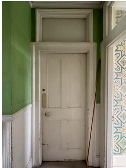
Figure 24; Modern fan lights above doors to Family Bathroom and Bedroom 3.
