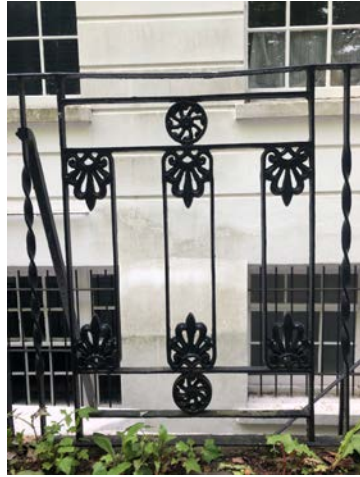
Figure 13: Painted cast iron panels on existing South Front Area, to match.
