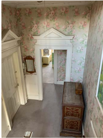
Figure 20: Modern painted timber overdoors on first floor landing
