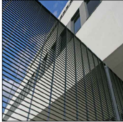
Welded steel mesh powder coated black
