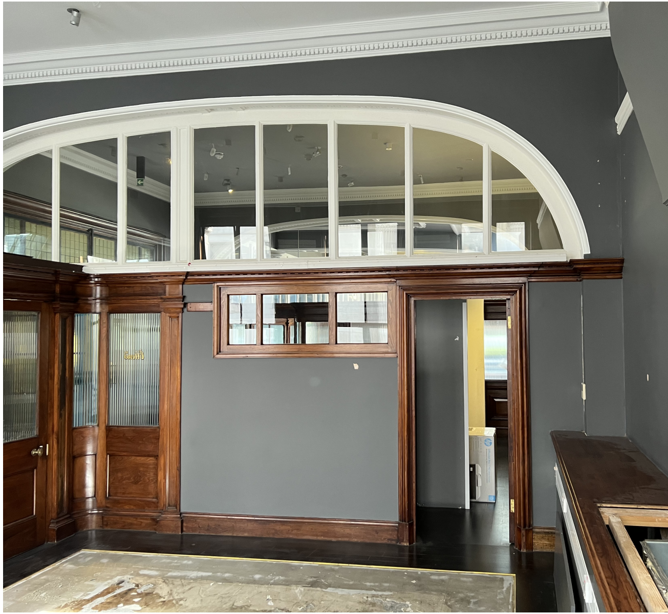
3 Existing photo; high level glazing to be removed
