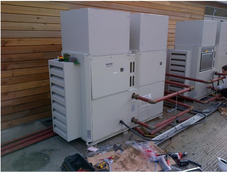
Figure 5 Indicative image of attenuator kit on VRF.
