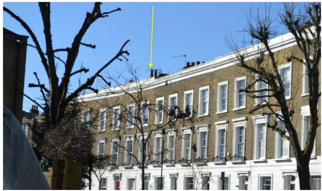
Figure 15: View of Grafton Crescent- No. 13 identified in yellow.
