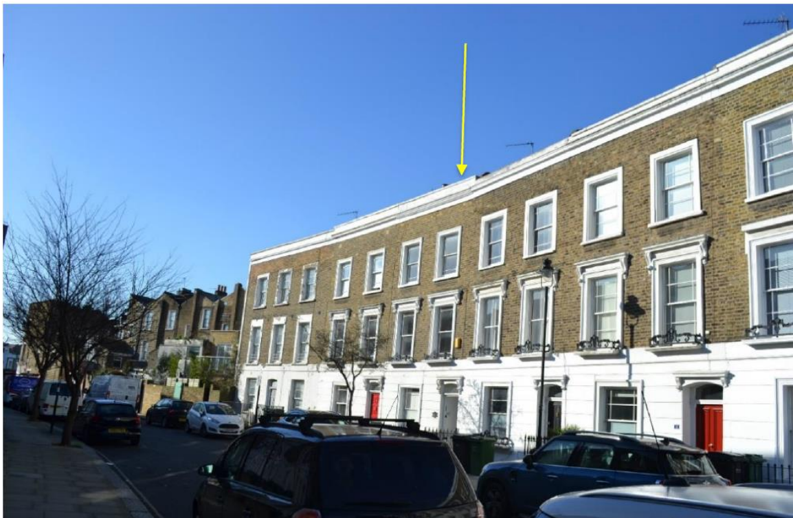
Figure 12: No. 13 Grafton Crescent identified by the yellow arrow.
