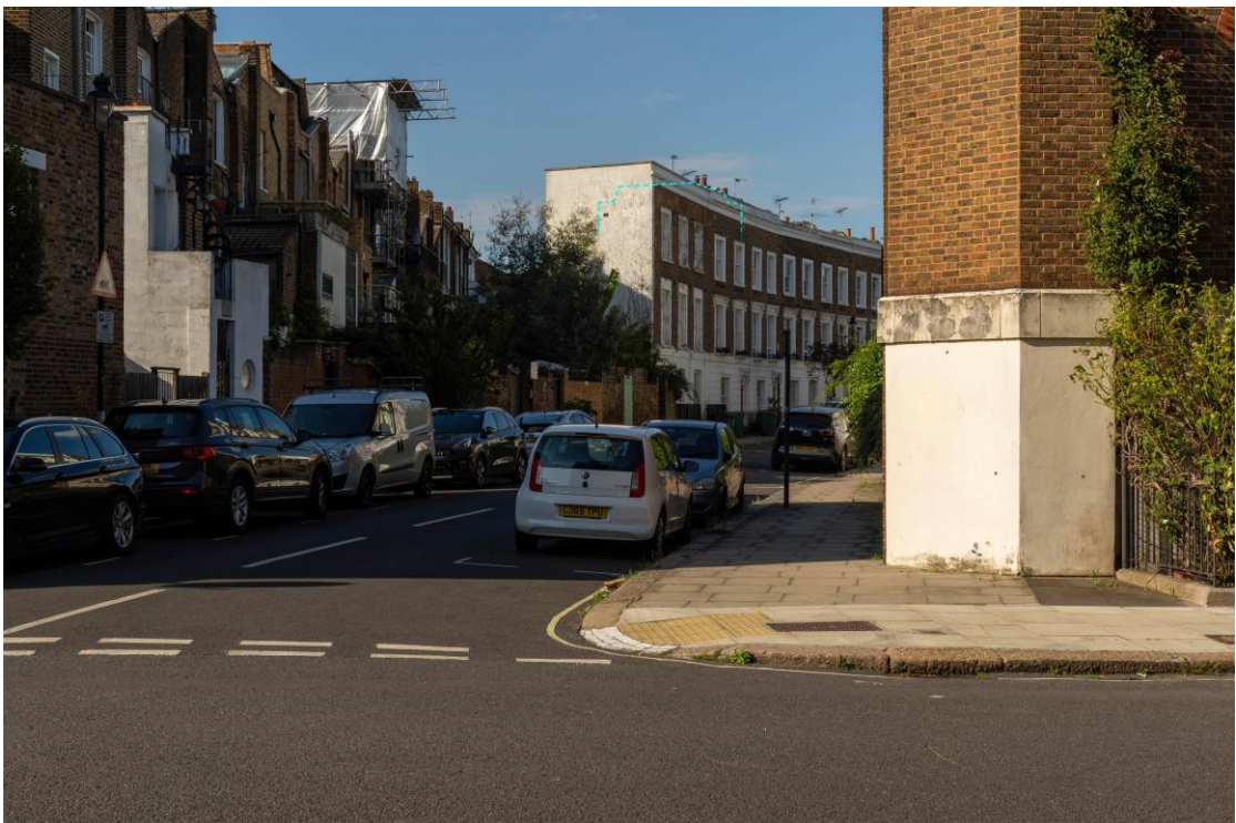
Figure 10: Verified Viewpoint 2, Castle Road opposite Grafton Crescent. Proposed mansard roof outlined in blue (OceanCGI, 2023)
