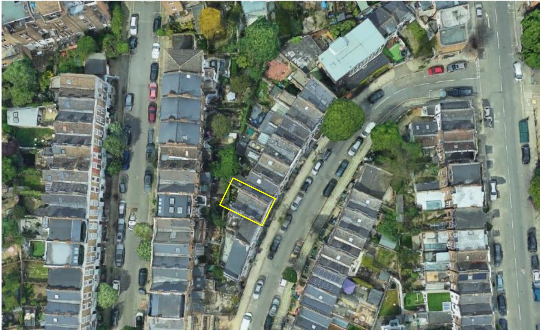
Figure 1: Aerial view of 13 Grafton Crescent - Site location highlighted in yellow.
