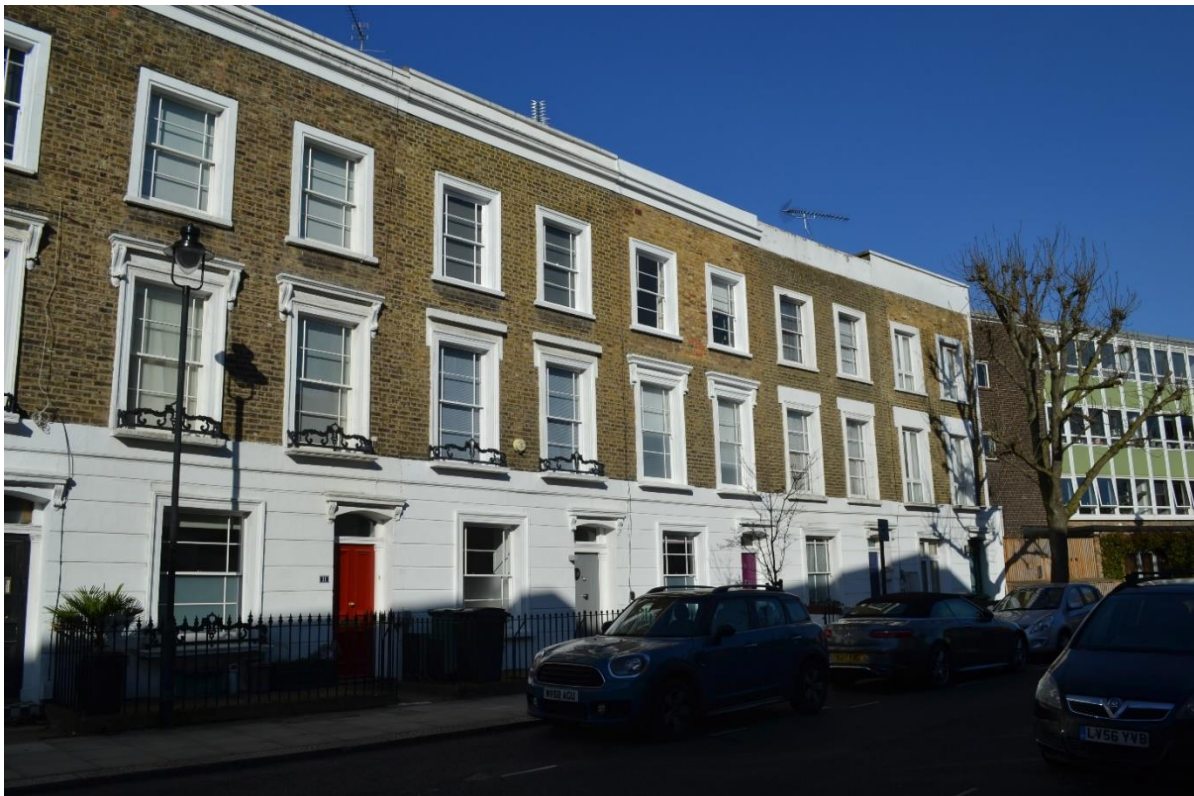
Figure 10: Front elevation of the terrace along Grafton Crescent looking north-east- No.13 not visible in the photograph.
