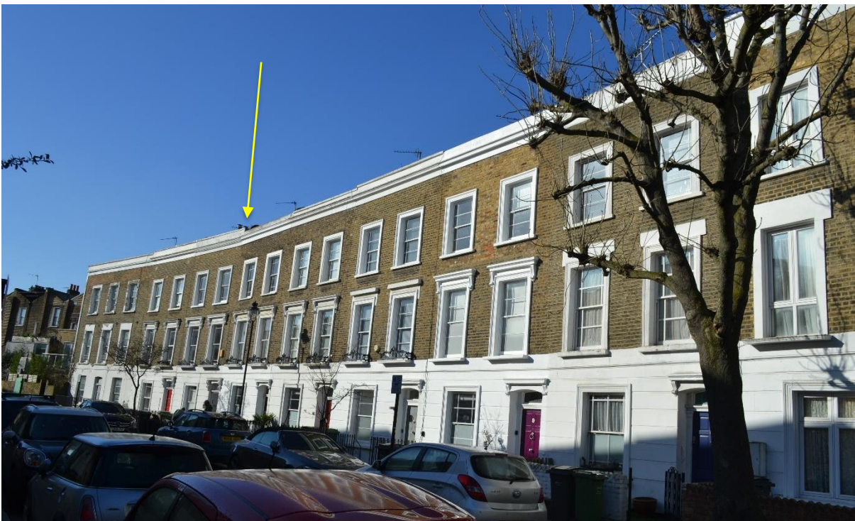
Figure 14: View of terrace along Grafton Crescent looking southwest- again note that roof is obscured from view due to the parapet and topography, only the top of the chimney pots are visible on No. 13 (highlighted in yellow).
