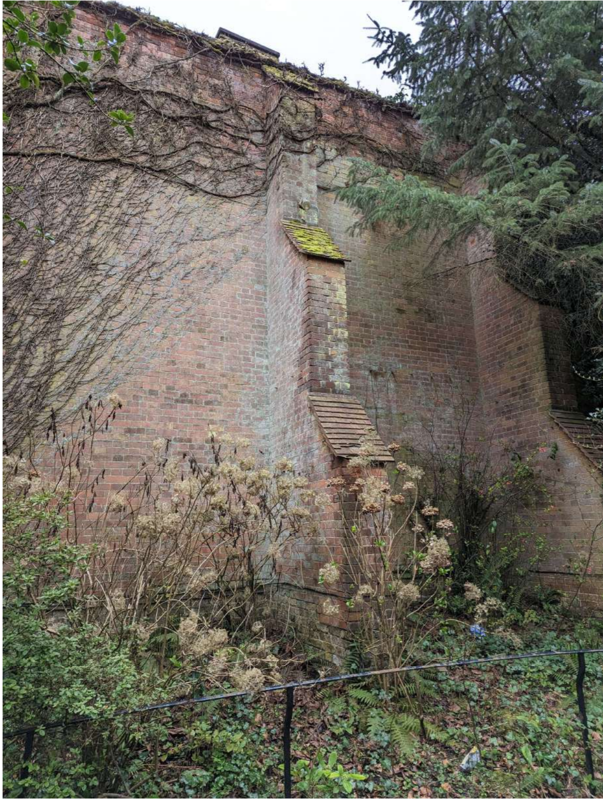
SOUTHERN BOUNDARY WALL
