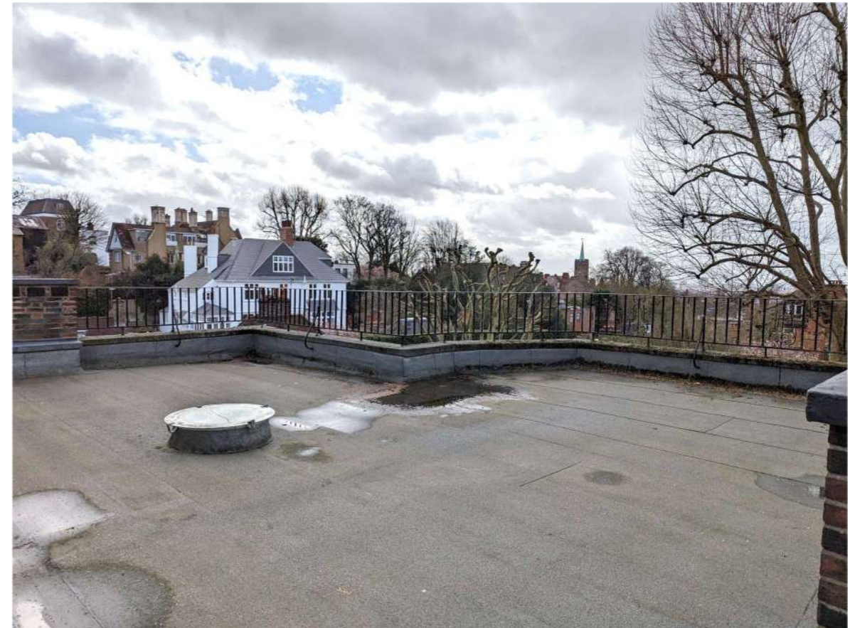
PHOTOGRAPH FROM EXISTING ROOF LEVEL, MAR 2023
