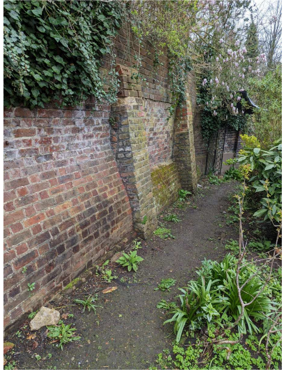
NORTHERN BOUNDARY WALL
