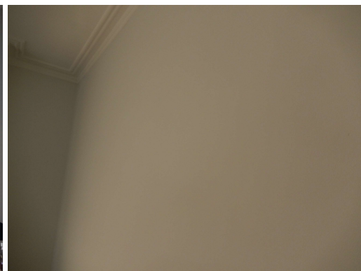
Spine wall - rear ground floor room
