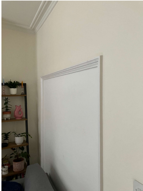
Spine wall - front ground floor room
