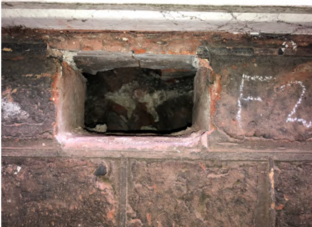
Figure 4.5 Intrusive investigation of front elevation exterior at First floor
