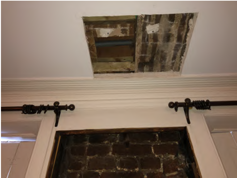
Figure 4.9 Intrusive investigation of floor structure at Ground floor
