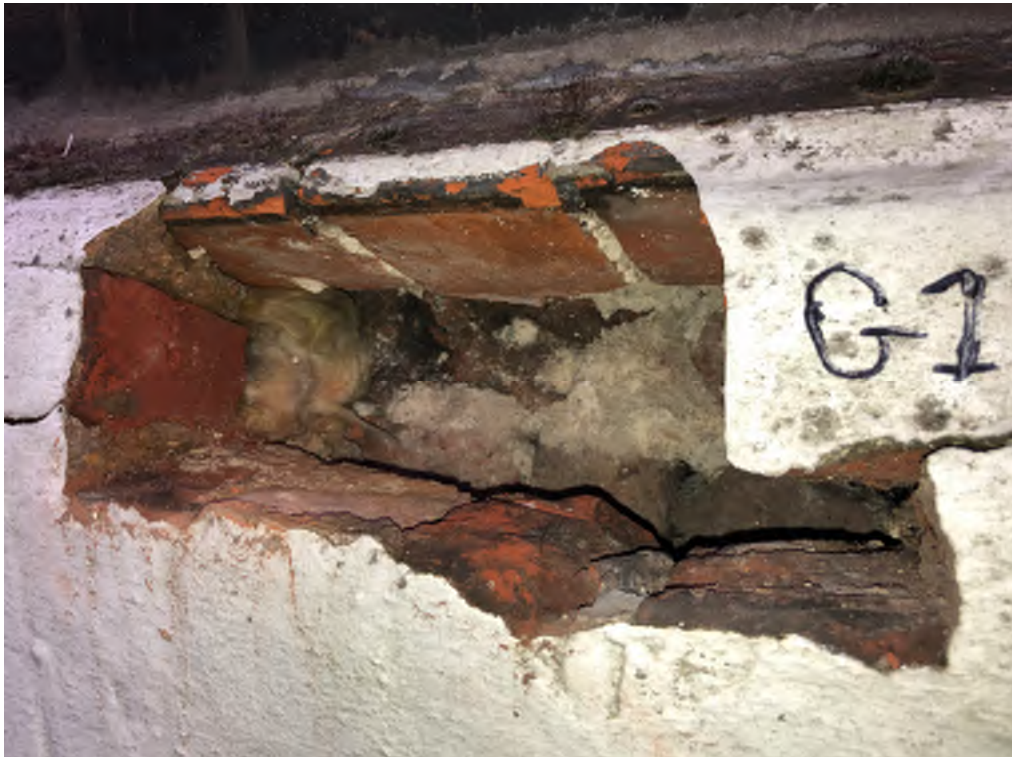
Figure 4.3 Intrusive investigation of front elevation exterior at Ground floor
