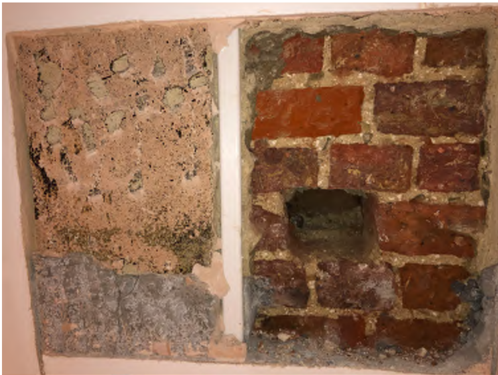
Figure 4.2 Intrusive investigation of front elevation interior at Basement
