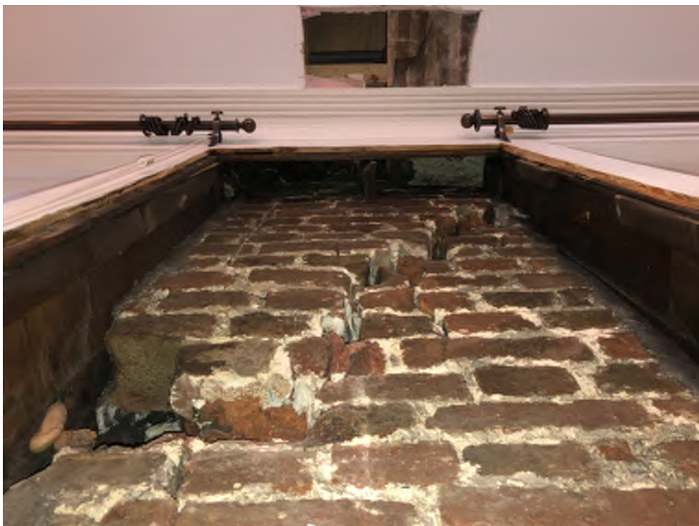
Figure 4.4 Intrusive investigation of front elevation interior at Ground floor
