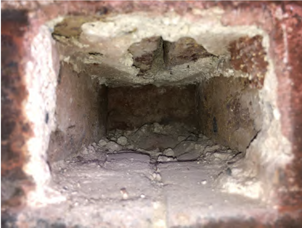
Figure 4.7 Intrusive investigation of front elevation exterior at Second floor
