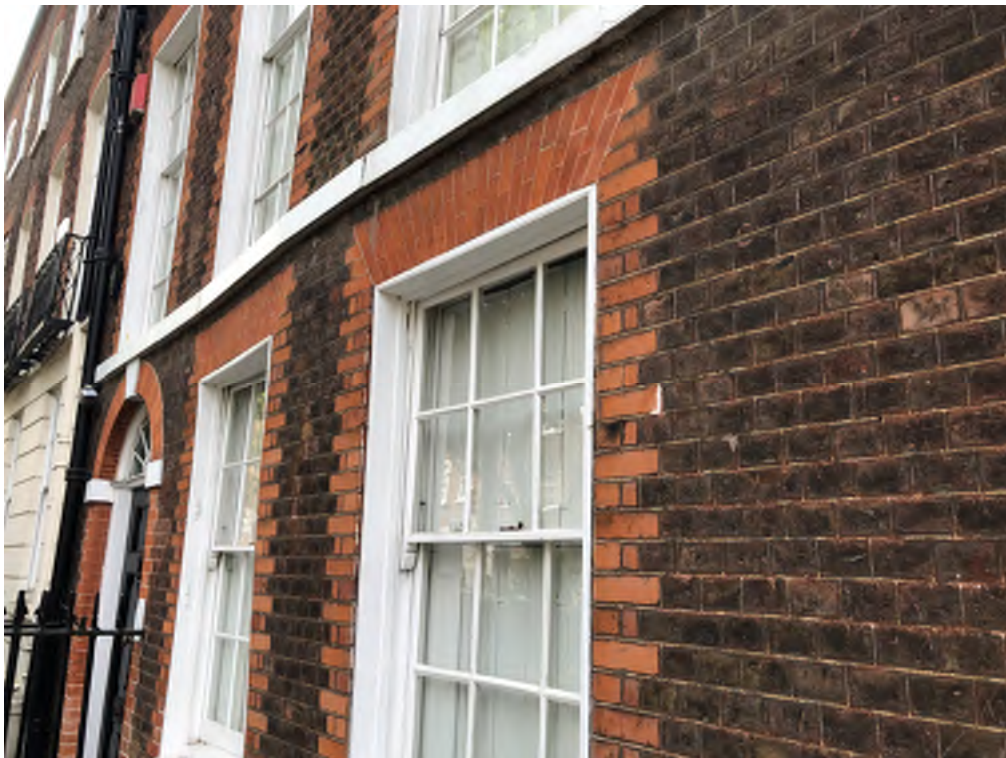
Figure 2.4 Close up view of front elevation
