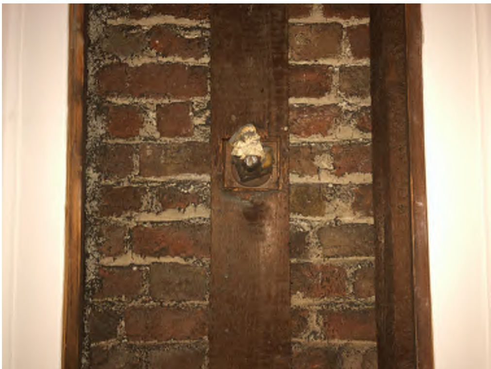
Figure 4.6 Intrusive investigation of front elevation interior at First floor
