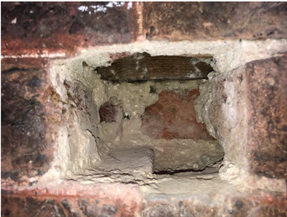
Figure 4.8 Intrusive investigation of front elevation exterior at Third floor
