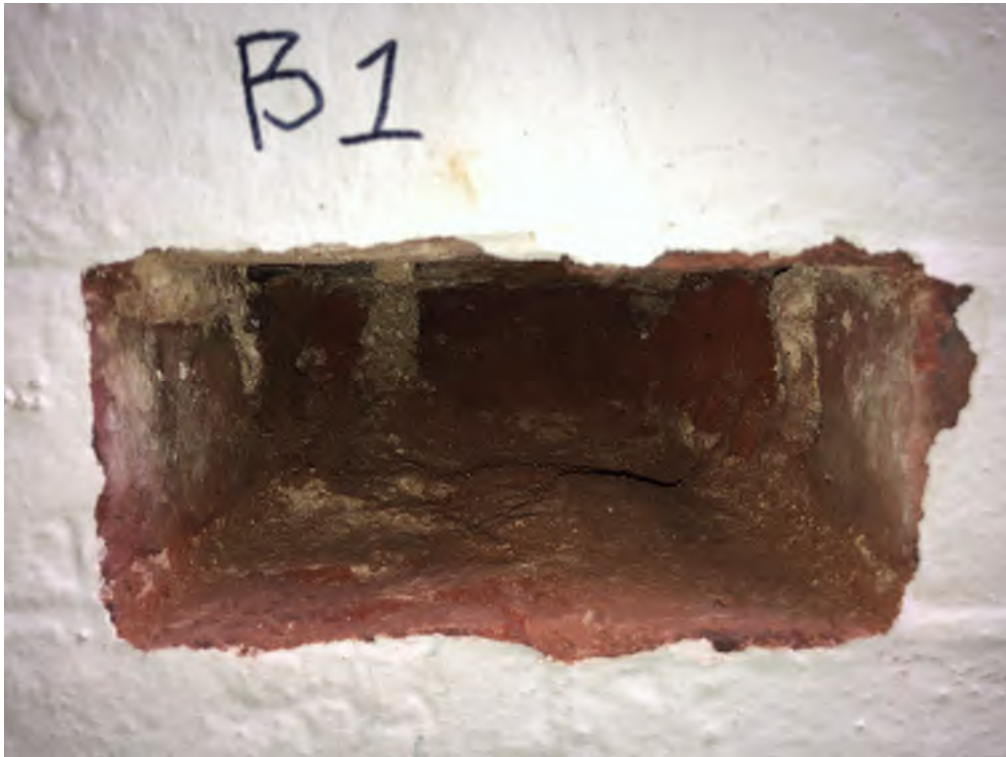
Figure 4.1 Intrusive investigation of front elevation exterior at Basement
