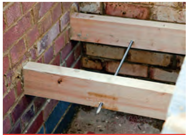
BowTie HDs installed through parallel floor joists
