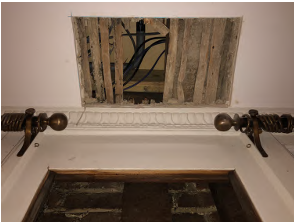
Figure 4.10 Intrusive investigation of floor structure at First floor
