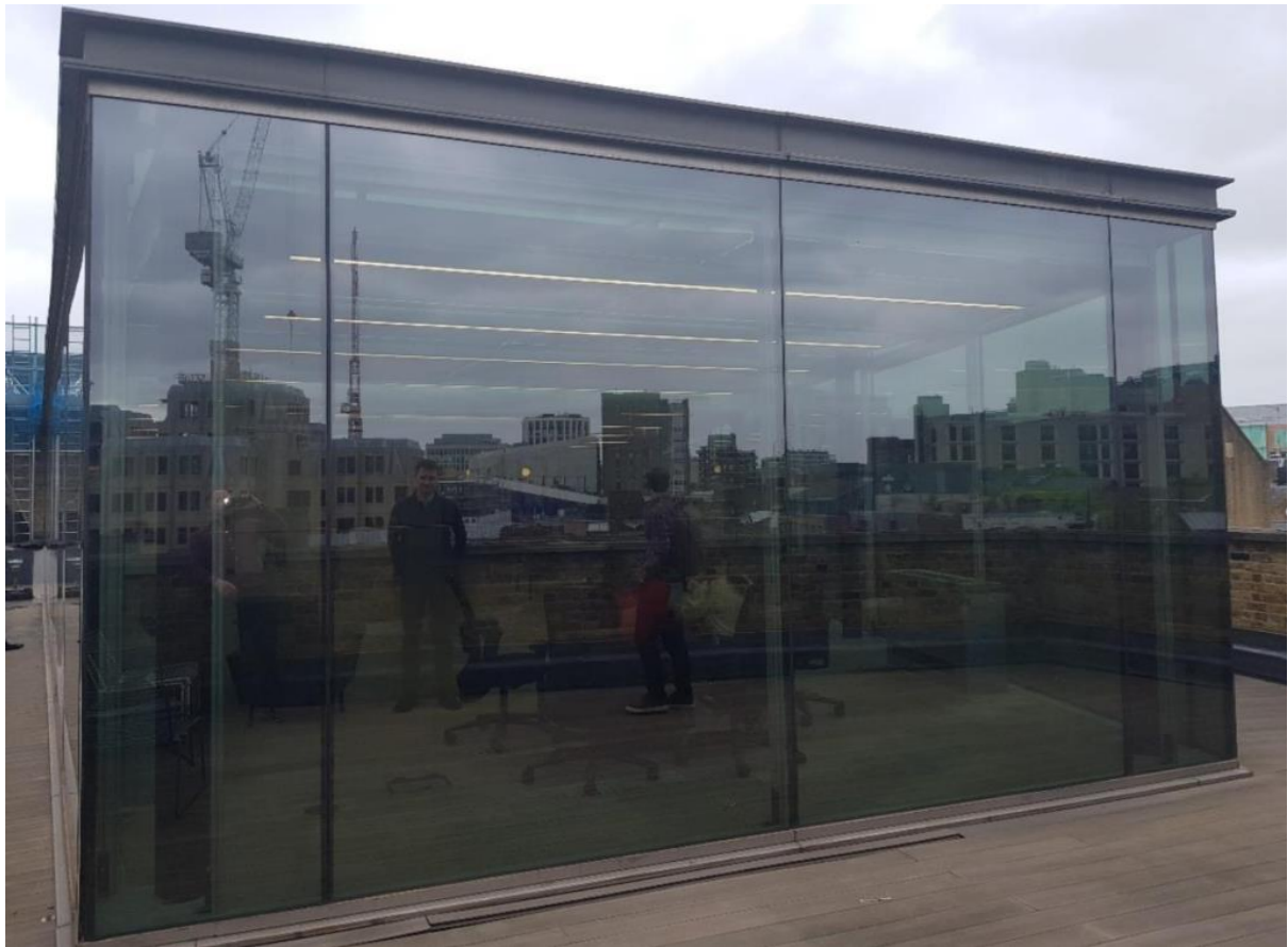
Figure 5 (above): Full height glazed windows now replaced by bi-folding doors
