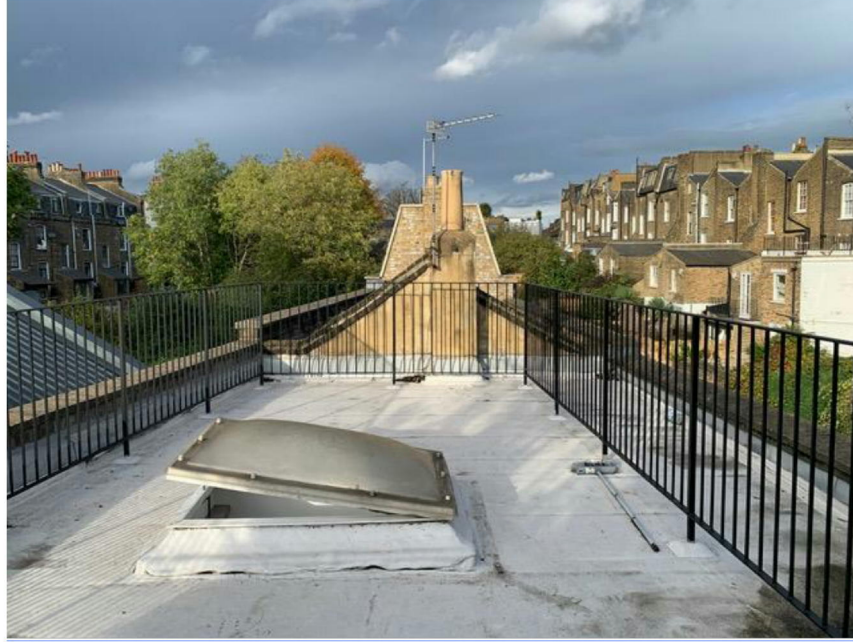
Photo 5 – Current Photograph of Railings (taken 31 October 2023)
