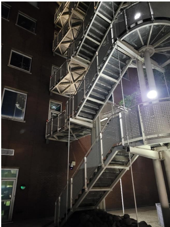
Photograph 3: High levels of lighting in the courtyard at night
