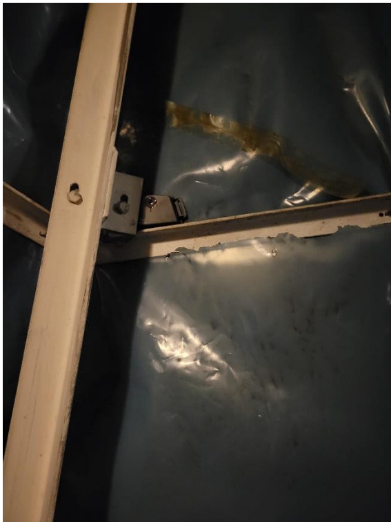
Photograph 2: Static detector deployed within the parapet/roof voids
