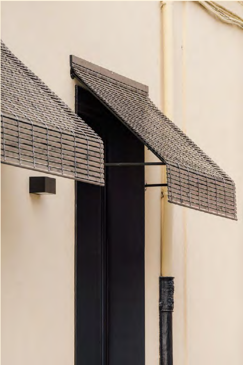
Upgrading the existing building fabric and providing a high level of insulation to the new facade elements and implementing simple passive design methods, such as awnings on the facade, will result in a refurbishment that is very low-carbon in operation
