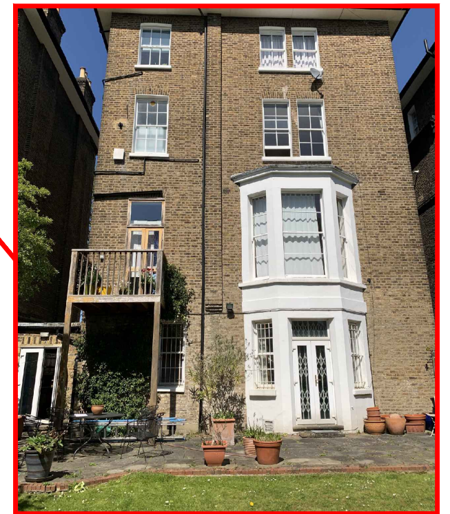
Existing 133 King Henry's Road Rear Elevation
