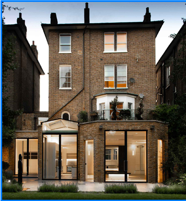
Approved Planning Application ref: 2010/0533/P dated 07.04.10 for 'Amendment to approved application 2009/2298/P (Erection of a side and rear extension to existing garden flat) to include erection of rear conservatory infill extension with glazed roof, modifications to rear patio doors and reduction in size of approved rear extension. of a double storey extension, single storey rear extension
