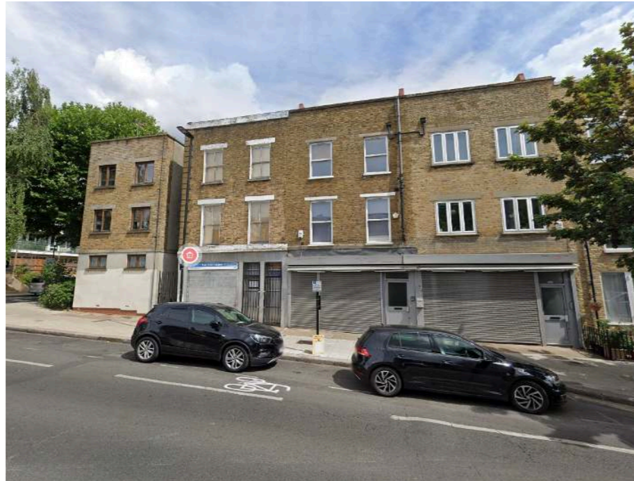
View to Front from Malden Road
