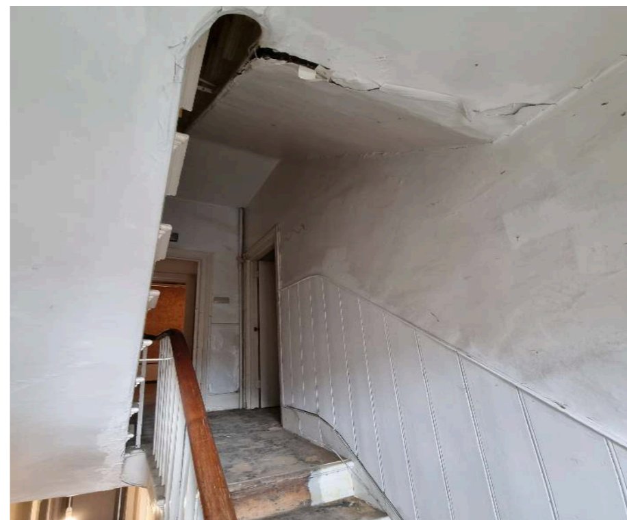
Hallway at the Property
