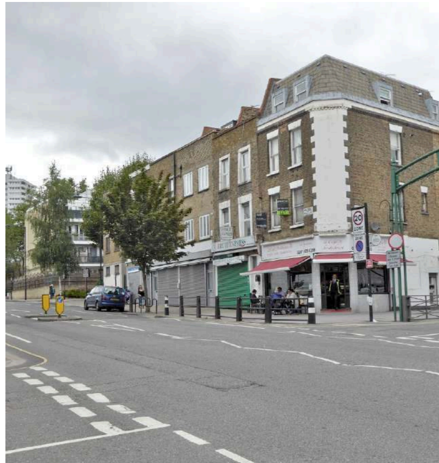
view of 118 -110 Malden Road and the corner of Queen's Crescent
