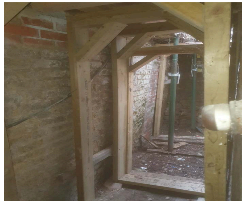
Structural Supports to the Front of the Property
